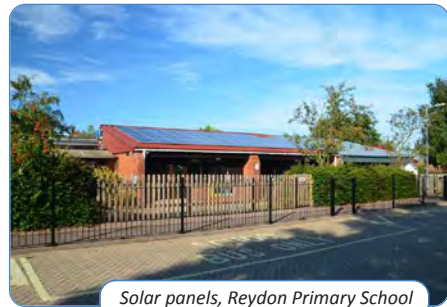
Solar panels, Reydon Primary School
