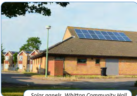
Solar panels, Whitton Community Hall
