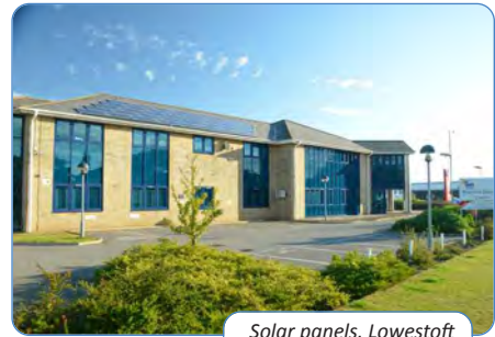
Solar panels, Lowestoft
