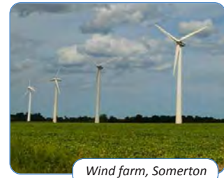
Wind farm, Somerton
