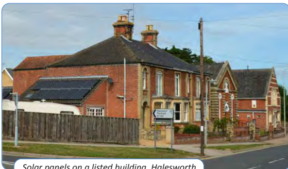
Solar panels on a listed building, Halesworth
