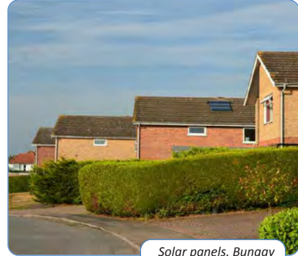
Solar panels, Bungay
