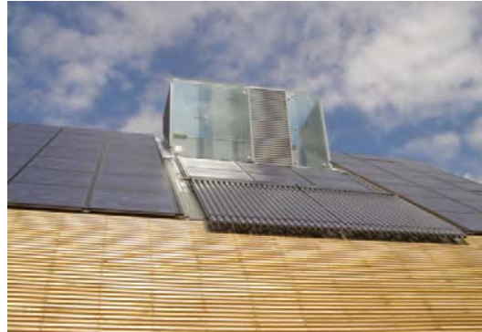
Solar panels on BRE demonstration home
