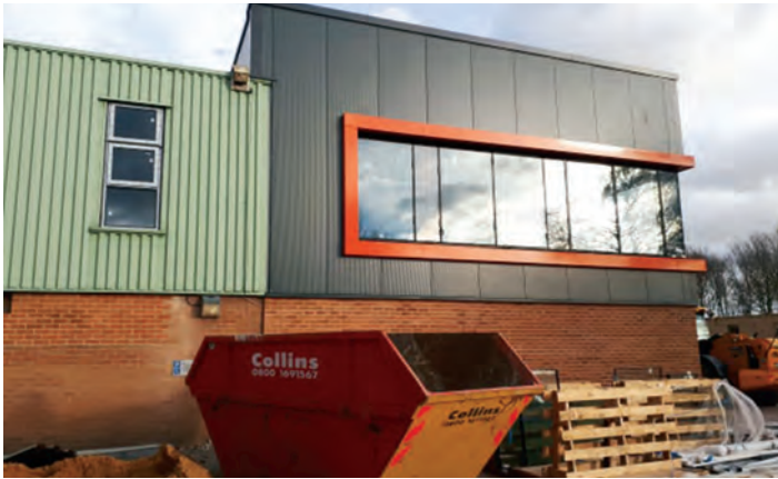
Work is well underway at Leiston Leisure Centre
