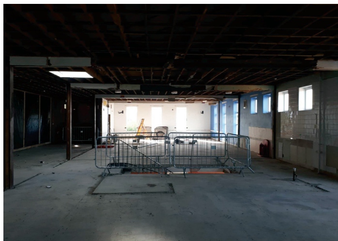
Work is well underway at Leiston Leisure Centre
