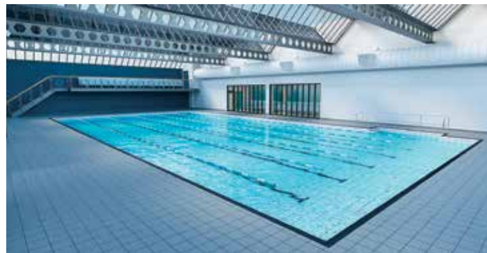
Refurbished swimming pool with a new viewing area
