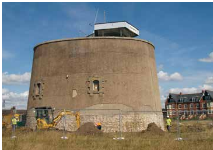
Martello Tower during refurbishments in August 2014
