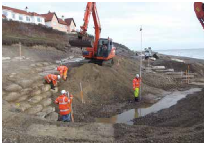
Work carried out at Thorpeness in 2011 - now a new plan is being considered for the coast here
