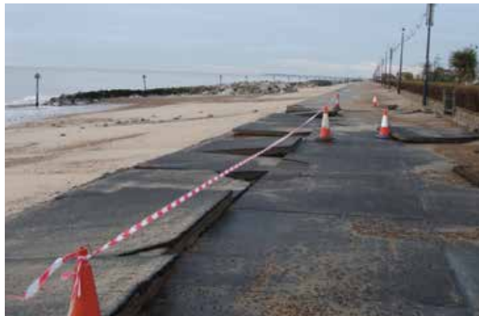
Storm damage to Felixstowe promenade
