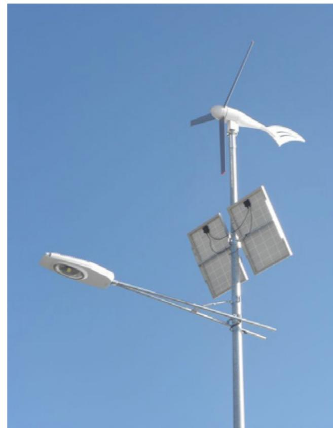
The use of renewable energy will be integrated where ever possible into the infrastructure that supports the PowerPark. This will include the provision of mini-turbines and solar panels onto street lighting columns to power lighting during periods of darkness. Solar panels will also be applied to the roof of suitable buildings to help with reducing the direct carbon footprint of new buildings within the PowerPark.
