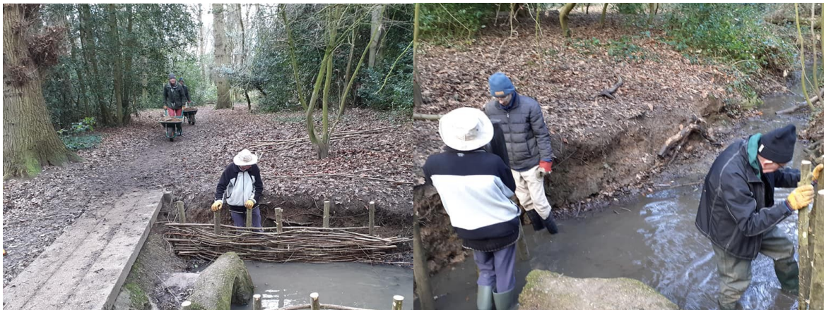
Reinforcing banks around an old bridge
