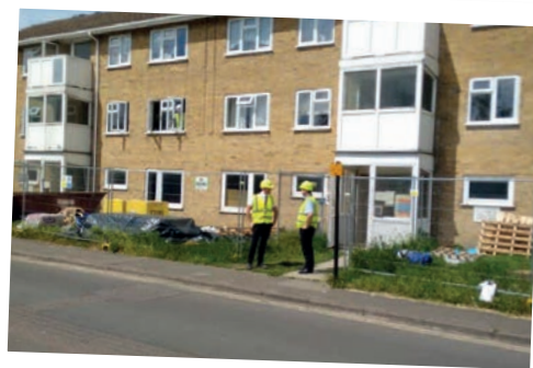
Britten House before refurbishment works commenced.
