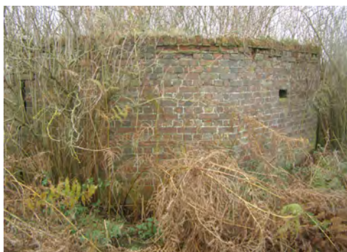
Eight sided brick built base to radio mast
