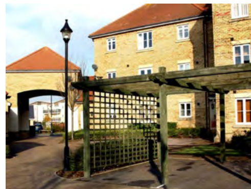
Rear courtyard parking with drive through access.
