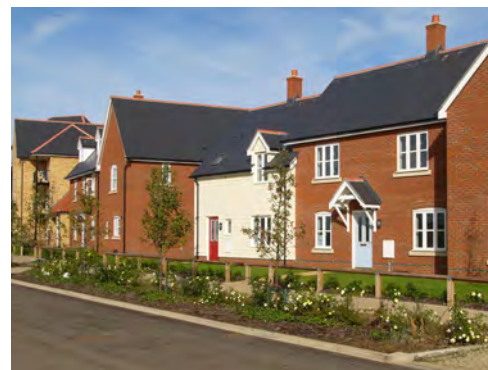
Varied roof planes and colour adds interest to street scene.
