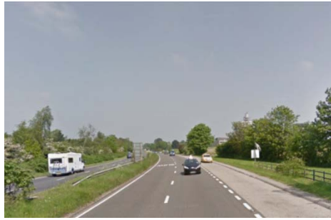
Figure 3: Southbound Carriageway looking North
