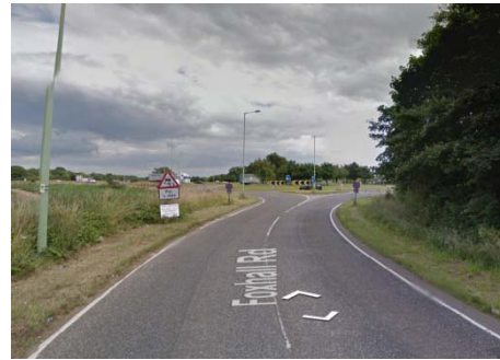
Figure 4: Foxhall Road (West) looking East
