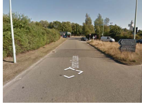
Figure 4: Barrack Square looking East towards Gloster Road
