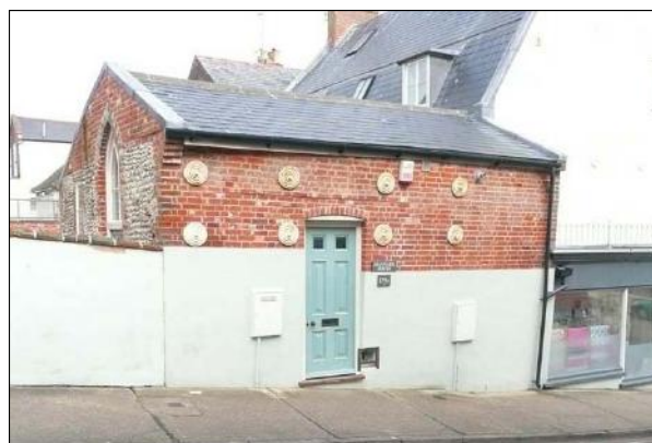
Brick walling with cast iron wall anchor plates, Choppings Hill
