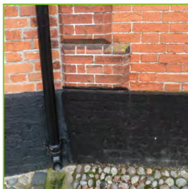
Brickwork quoins, cast iron downpipes and flint cobble surfacing in Northgate
