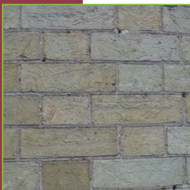
Mortar joints with a 'penny roll' in Hungate
