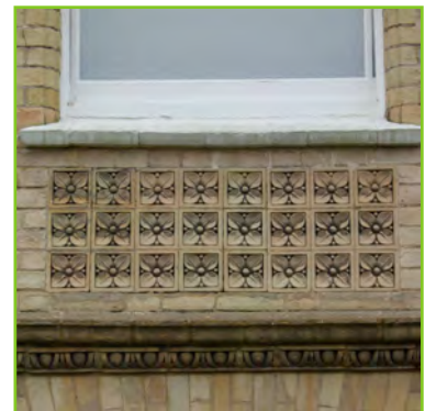
Moulded white brickwork in Station Road
