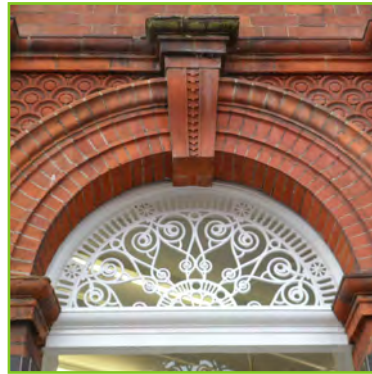
Moulded brickwork and cast iron in Smallgate
