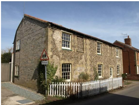
Nos. 1 & 2 Bridge Street
