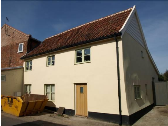
Rear wing of the former shop on the corner of Bridge Street and The Street
