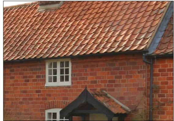
Brick on edge brickwork at The Anchorage.
