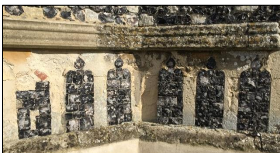
Flint flushwork panels to the base of the Church tower.
