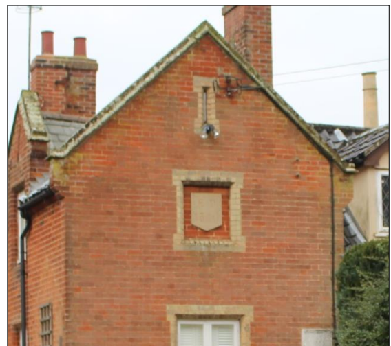
Red clay brickwork with gault brick dressings, to The Old School House.
