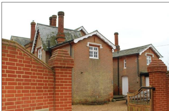
Extensive use of red brick to the Old Rectory, including to the rebuilt section of boundary wall and gate piers.
