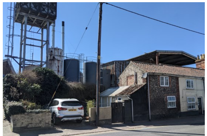
The printing works from Broad Street
