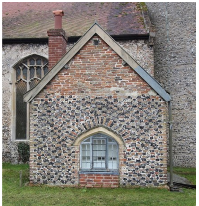
Right: Decorative brick and flint work, Holy Trinity Church Vestry
