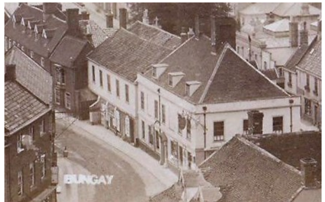
The Three Tuns and its assembly rooms c1920
