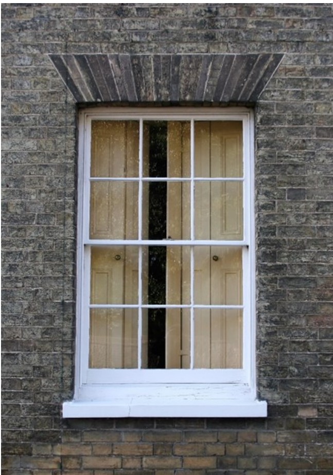
A ‘hornless’ sash window of twelve lights, Upper Olland Street, possibly early nineteenth century.
