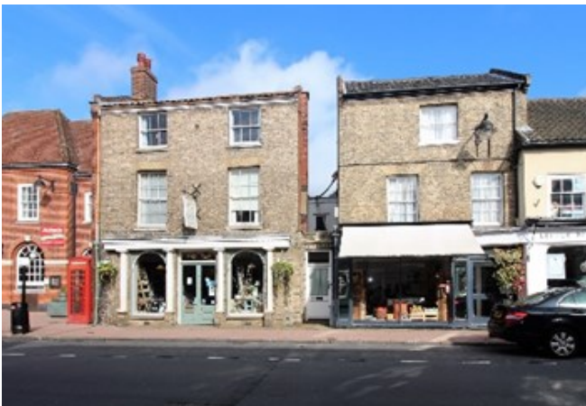
Left Top: Pale red brick, with ‘rubbed’ brick used for the lintels, Trinity Street, mid to late eighteenth century remodelling of a seventeenth century house.
