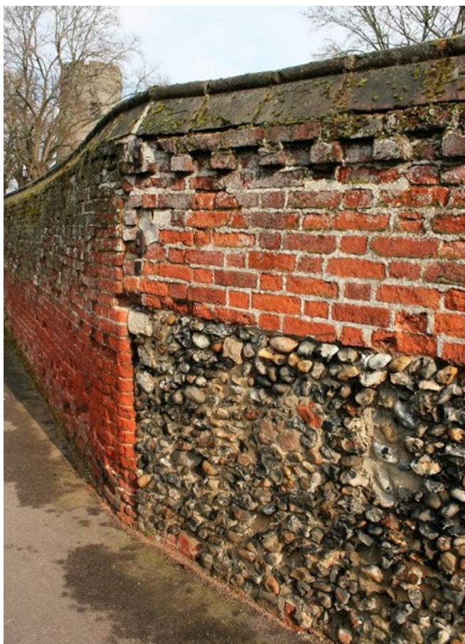
Left Top: Flint rubble and later red brick to boundary wall Trinity Hall, Trinity Street
