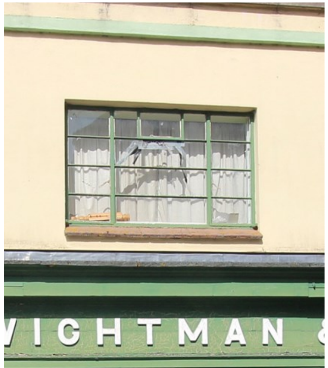
Right: 1930s metal framed casements, Wightman’s Building, Cross Street
