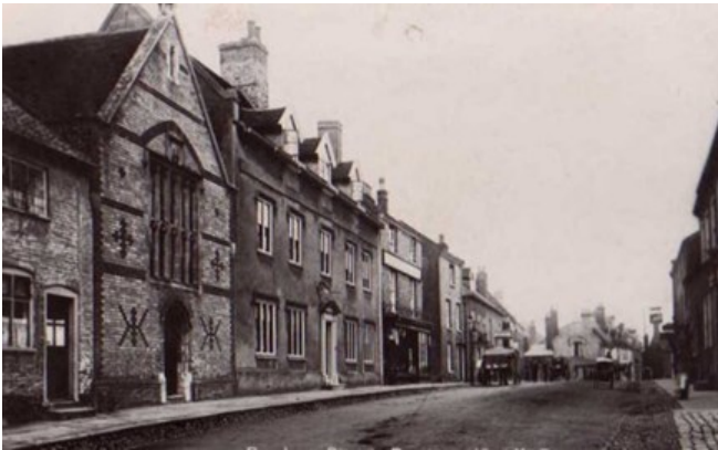
The former Grammar School, Earsham Street (Demolished)
