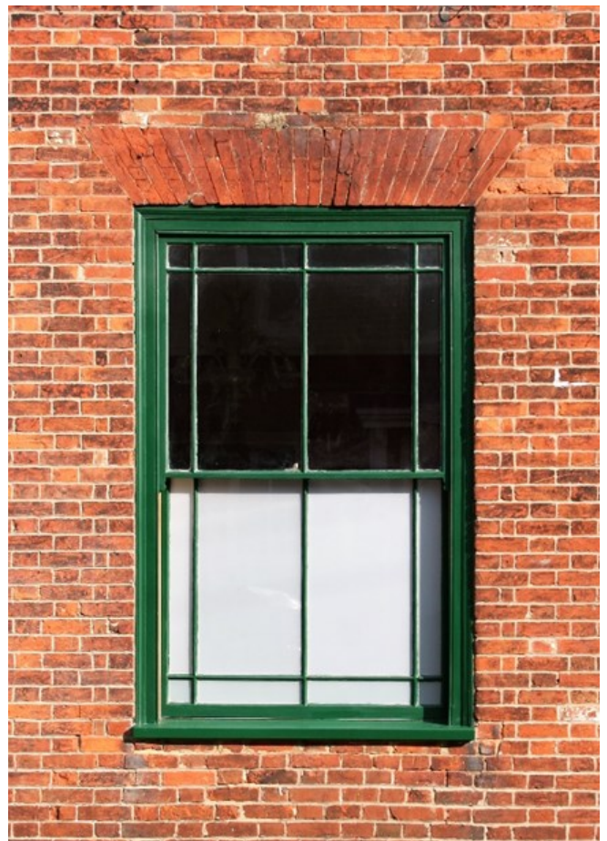
A ‘horned’ sash window with margin lights and a fine rubbed brick lintel, Broad Street, probably of mid-nineteenth century date.
