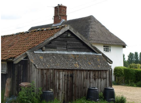
Black weatherboarding and Pantile
