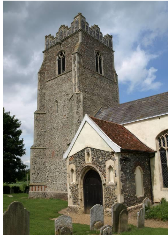
St Peter's Church Tower
