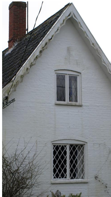
Overpainting of brickwork
