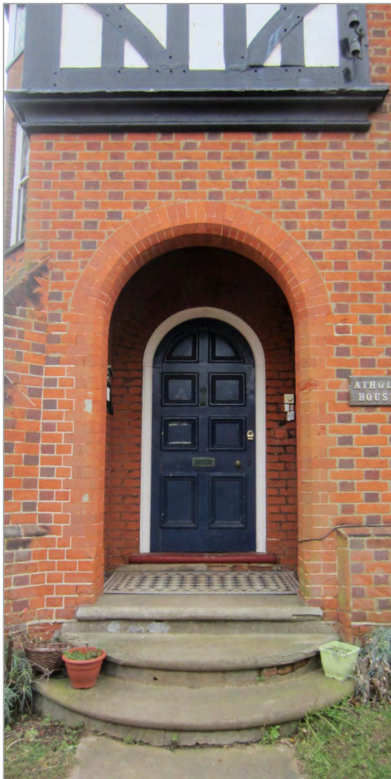
Half-timbering, burnt headers, quality joinery, decorative tiling
