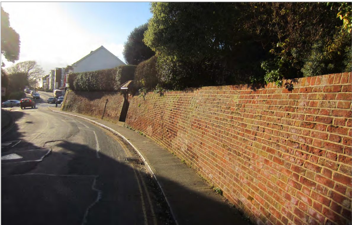
Battered retaining garden walls are a feature at the west end of Hamilton Gardens
