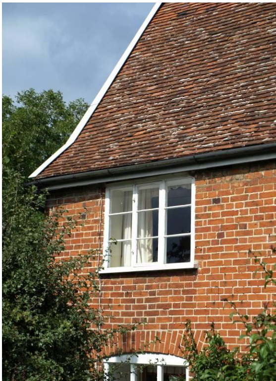
Red brick and plain tile roof covering
