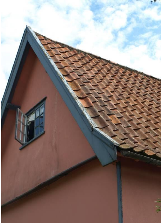
Painted render and pan tile roof covering
