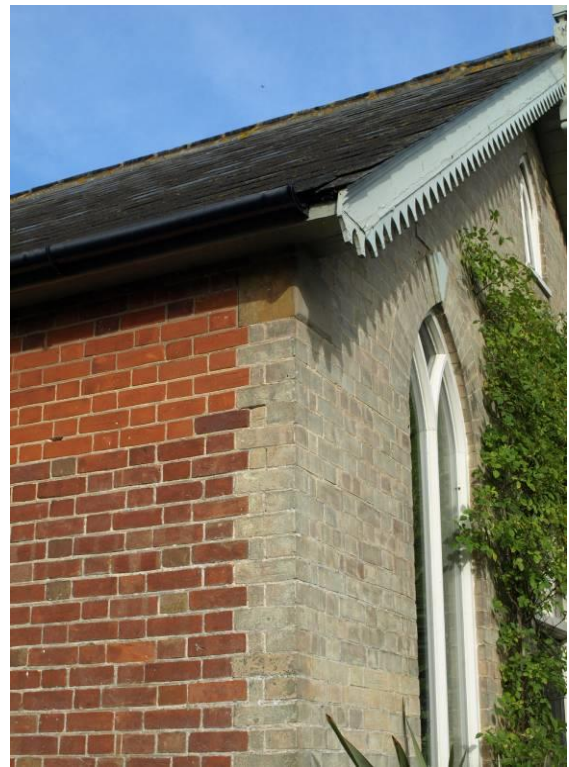
Suffolk cream or gault bricks with slate roof covering
