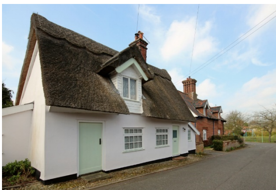
Figure 36: Thatched Cottage from the south
