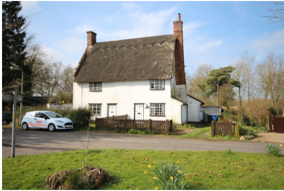
Figure 15: Vernacular materials, such as render and thatch, commonly found to smaller cottages clustered around The Green
