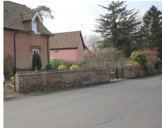
Figure 18: The important visual contribution well-detailed boundary walls make to the streetscape
