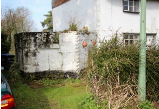
Figure 50: Pillbox attached to Greenview
