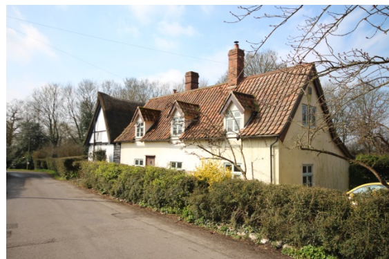
Figure 13: Red clay pan tile coverings replacing thatch to roofs of older cottages
