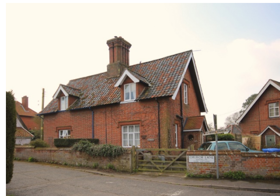
Figure 38: Church Lane elevation of Nos. 63-67
