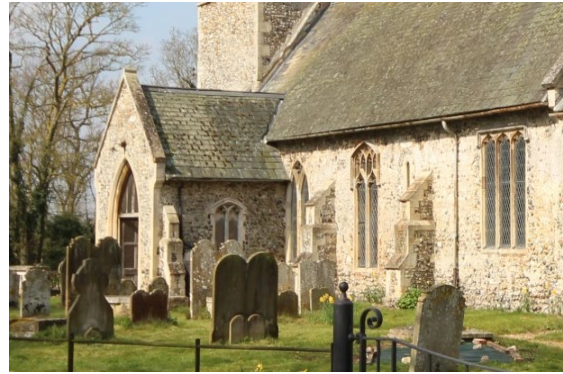
Figure 12: High quality materials, such as stone, flint and slate, reserved for higher status structures and detailing
