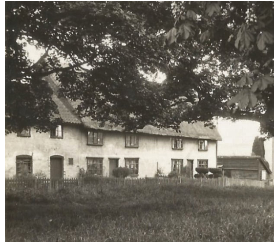
Figure 52: Nos.82-83 The Green c1920, showing now demolished outbuilding to its north.
