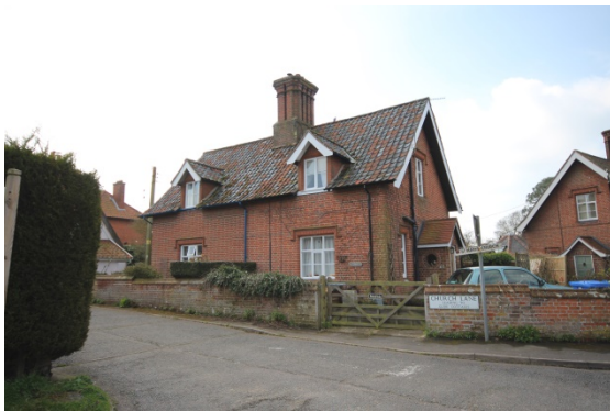
Figure 16: Black glazed pan tiles and finely detailed brickwork, denoting a relatively high-status property
