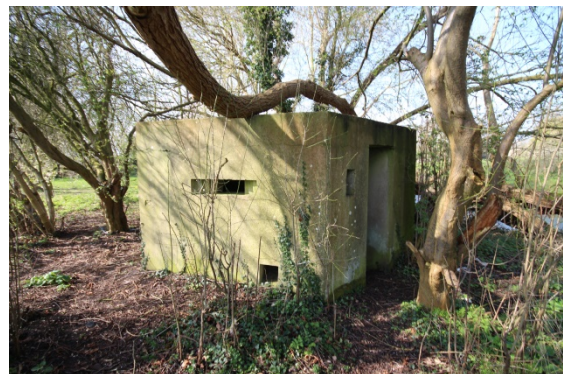
Figure 14: The use of shuttered concrete to a pill box. Other uses of this material exist to anti-tank cubes and the Grade II* bridge over the River Waveney
