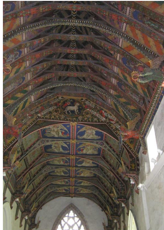
St Mary's Church Roof
