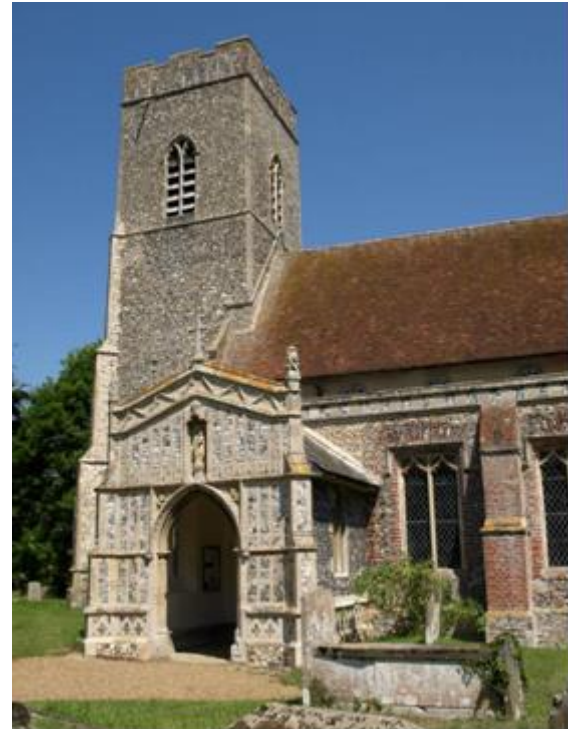
St Mary the Virgin Church Tower
