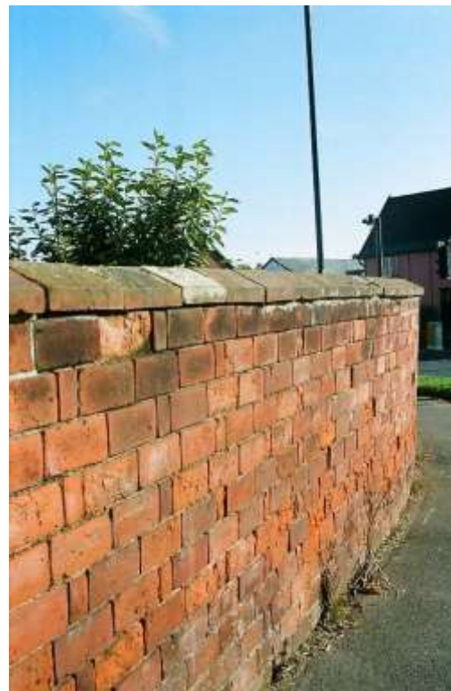
Rat-trap bond red brick boundary wall
