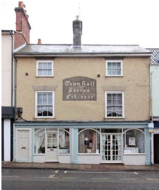
C2003 shop fronts at Nos.43-44 High Street
