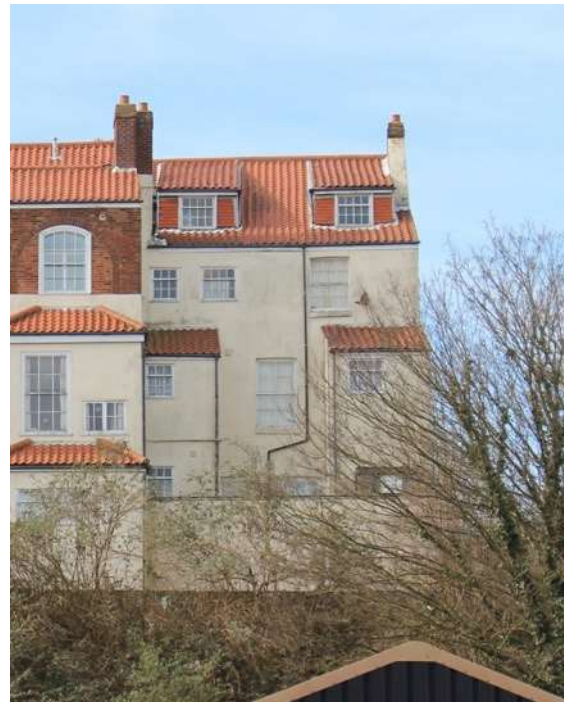
Rear elevation of No.2 High Street from Whapload Road
