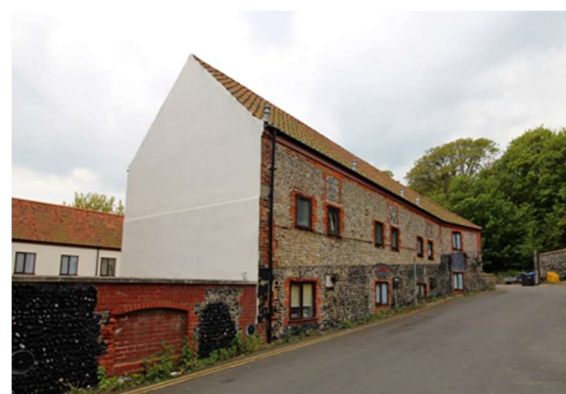
The use of flint, red brick and render at No's 14 to 17 'The Anchorage', Whapload Road
