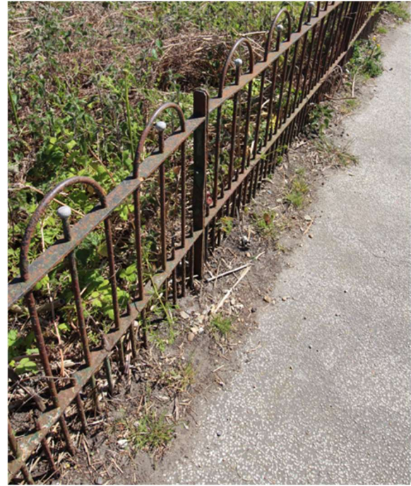
Decorative iron railings
