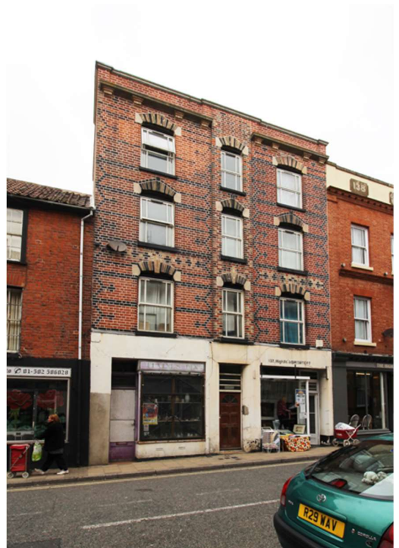
Polychromatic brickwork
