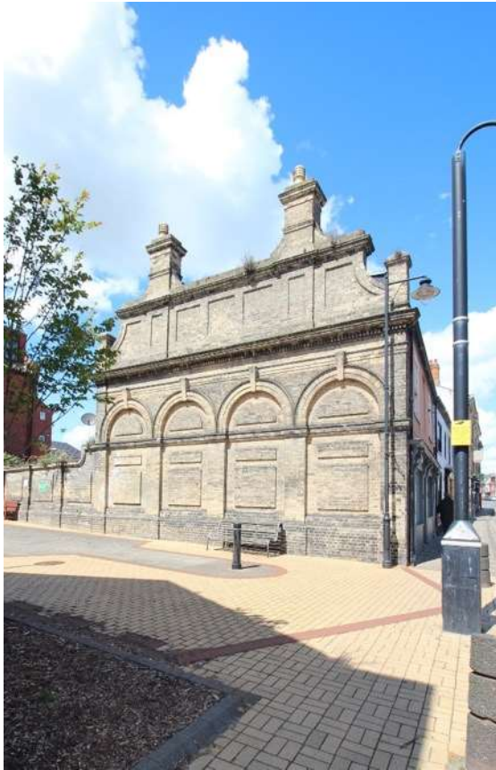
Return elevation of No.147 High Street
