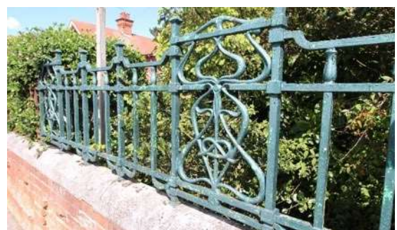
Railings to former gardens of Briar Clyffe, Corton Road
