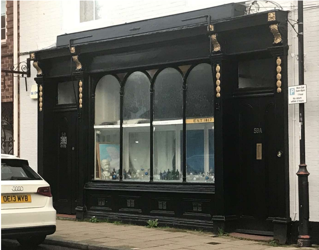
No.59 High Street, a rare and unusually fine surviving example of a chemist shop of c1851. Listed at Grade II.
