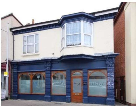
No.178 London Road North
