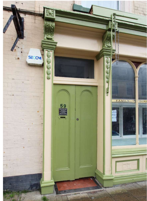
High Quality Shopfront at No.59 and 59A High Street
