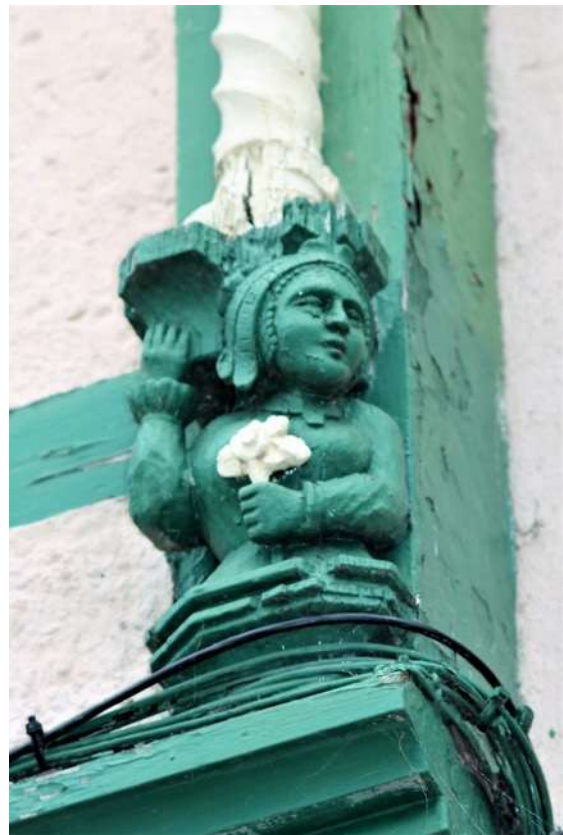
Detail of Nos.90-91 High Street designed by William Oldham Chambers for Adam Swallow Clarke c1880.
