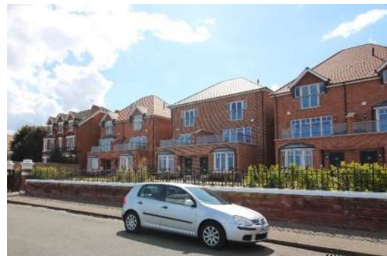
Early twentieth first century housing on Gunton Cliff
