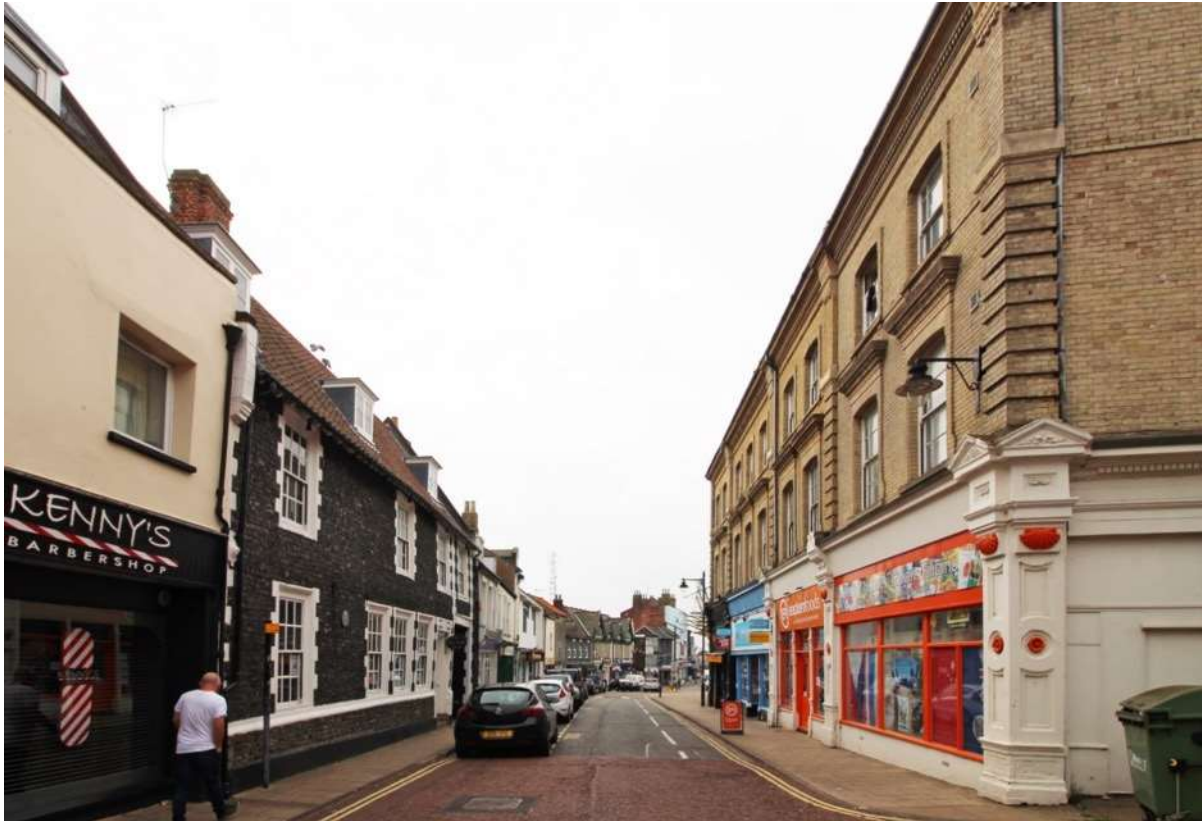
Looking South on the High Street from the corner of Old Market Street, the substantial building on the right was built for John Devereux as a grocery and provisions store.
