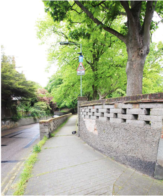
Cast concrete walls and balustrades
