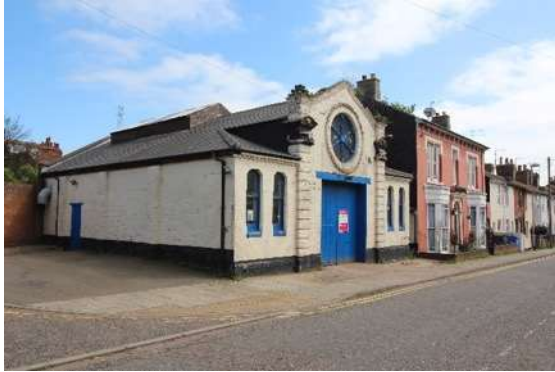
AP Motors, Former Drill Hall, Arnold Street
