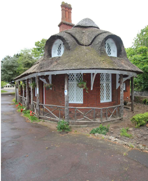
Thatch with tree trunk columns (cottage orne)
