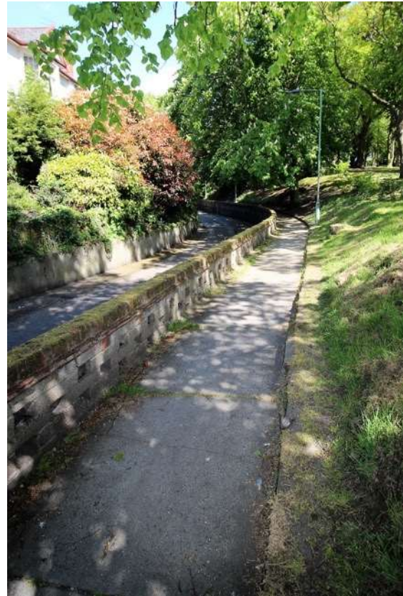
Retaining wall to The Ravine
