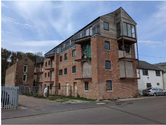
No. 312 to No. 314 (inc), Whapload Road, under conversion.
