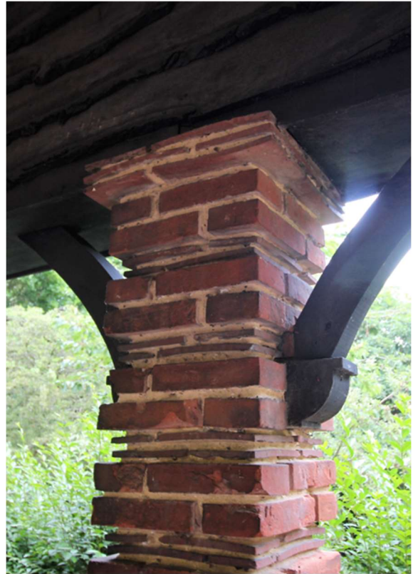
Tile and brick column detailing
