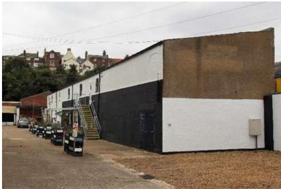
No.231 Whapload Road, northern block
