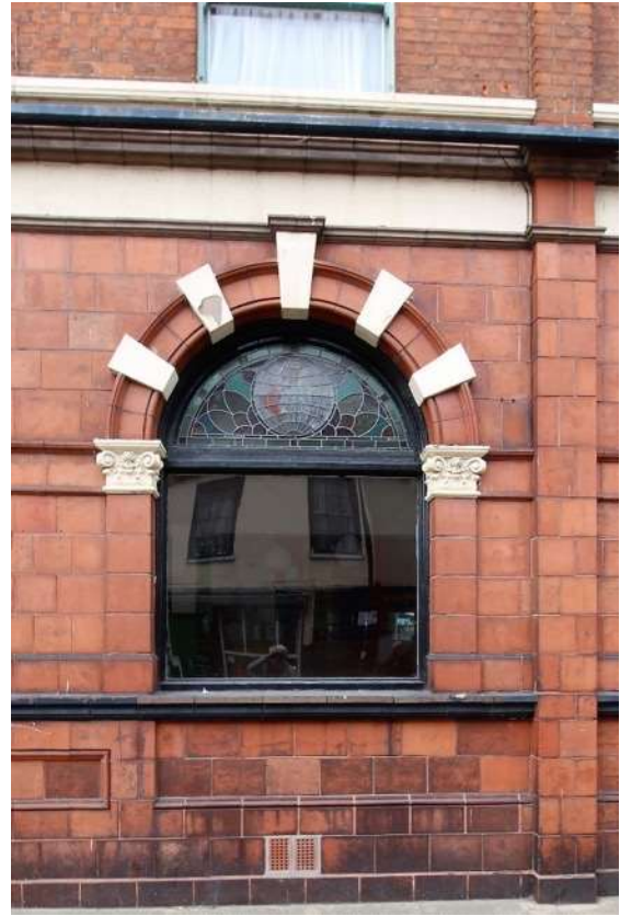
A typical window, at the former New Globe Public House, No.131 High Street, showing stained glass of c1905 depicting a globe.
