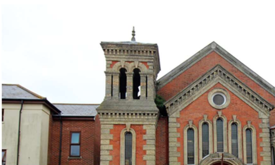
Campanile to the United Reform Church, London Road North
