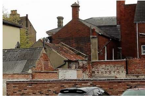
Cobble outbuilding to rear of The Old Blue Anchor
