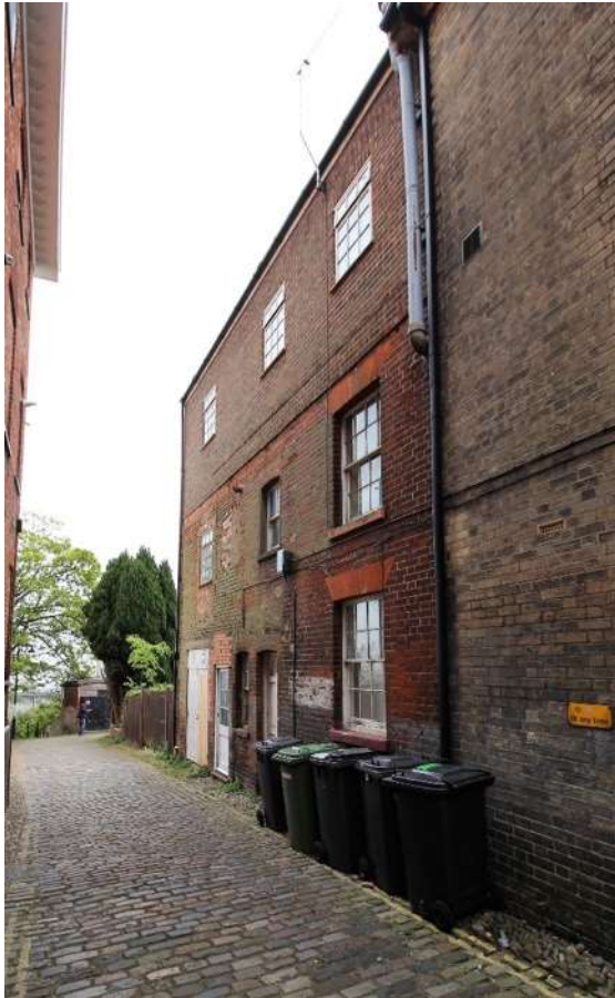
Former Cottages at the High Street corner of Crown Score
