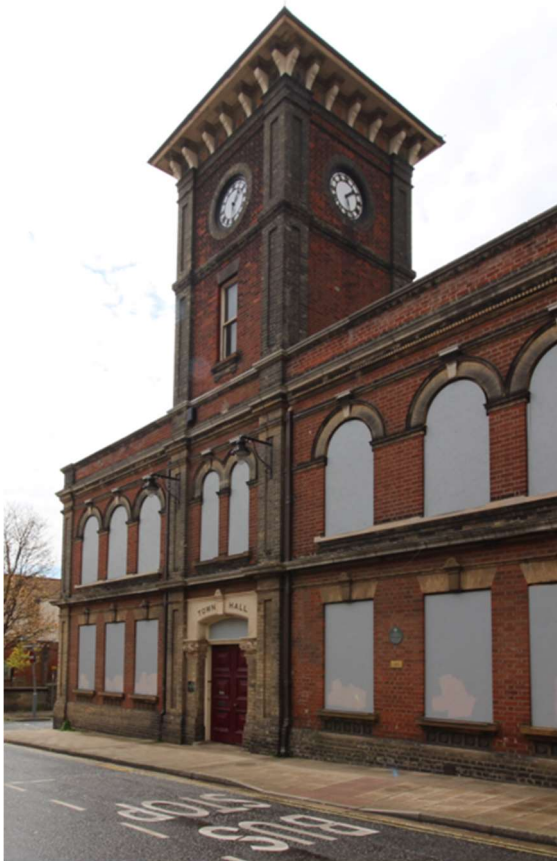
Empty Grade II Listed former Town Hall, High Street
