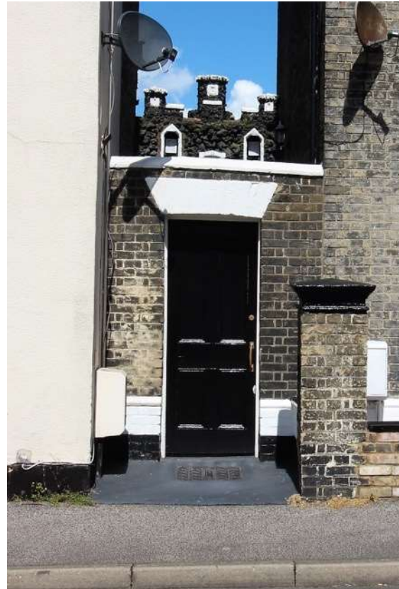
Gate at No.38a, Crown Street West
