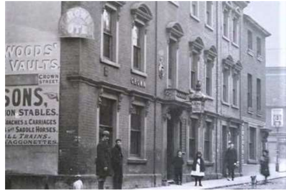
No.152 c1890 before loss of original ground floor section of façade.
