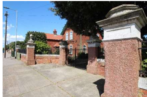
Gate piers to south of No.30 Corton Road
