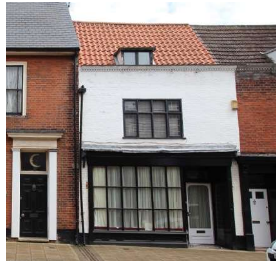
No.31 High Street, now a house, the small pane glazing was inserted into a later nineteenth century shop front c2002.
