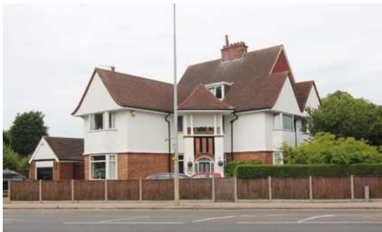
An arts and crafts villa on Corton Road designed by RS Cockrill now with unsympathetic replacement windows.
