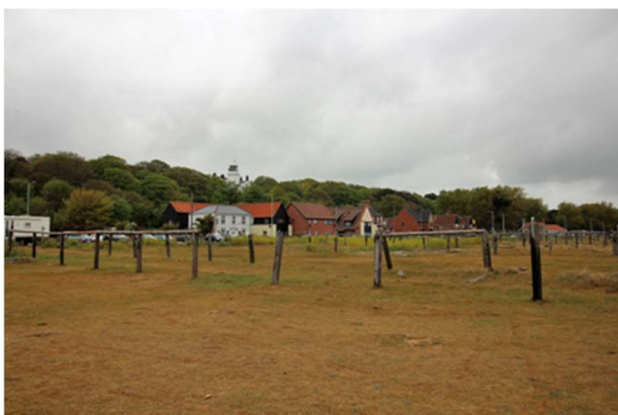
The Net Drying Ground, looking north west The structures on the net drying ground, while interesting and illustrative, are of modern
