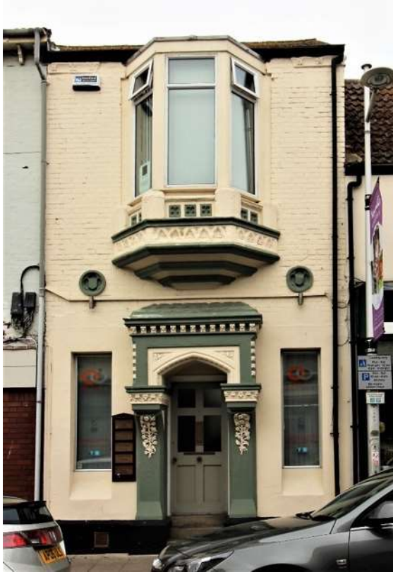
No.167 London Road North
