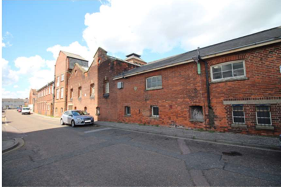
Crown Brush Factory, Crown Street West (Factory Road elevation)
