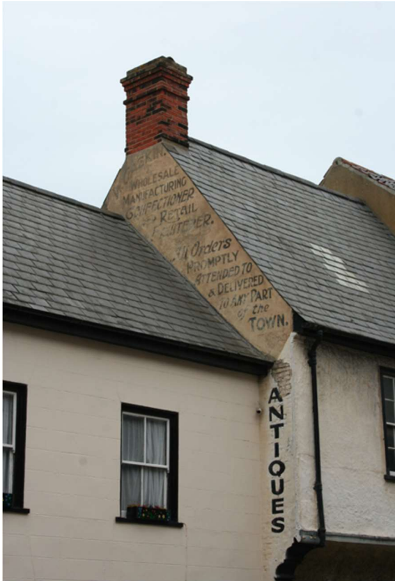
Slate roof covering
