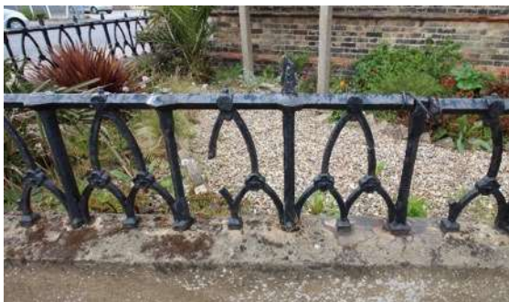
Railings around north and east sides of Christ Church
