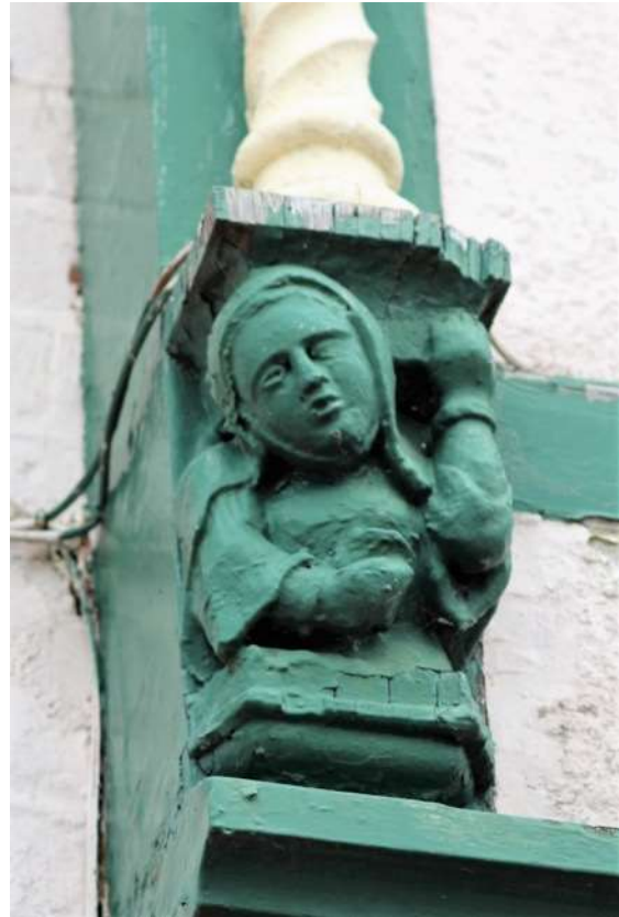
Detail of Nos.90-91 High Street designed by William Oldham Chambers for Adam Swallow Clarke c1880.
