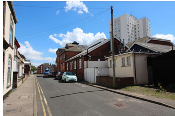
View looking east along Crown Street West
