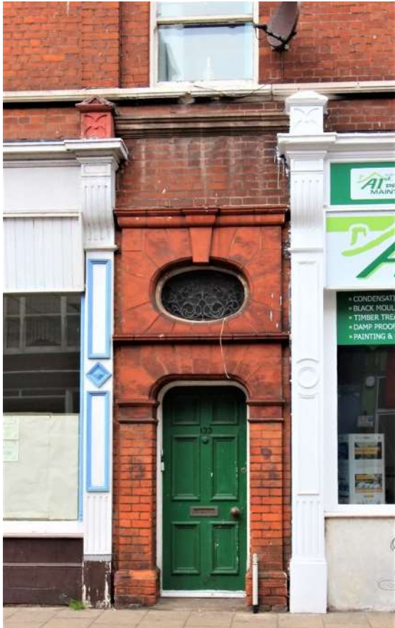
Doorway, No.133 High Street
