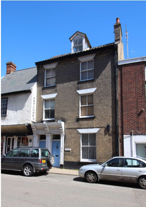
Suffolk white (or gault) brickwork
