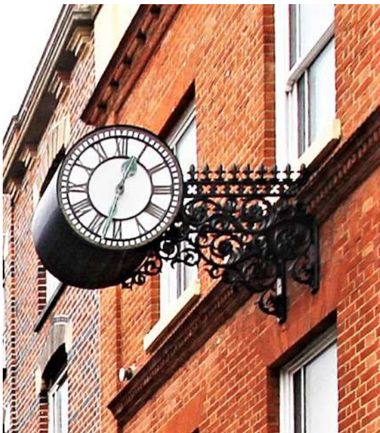
No.138 High Street clock installed c1888 probably to advertise the watchmaking business of Edmund Crake.
