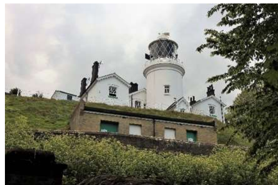
Storage building at High Lighthouse, Yarmouth Road
