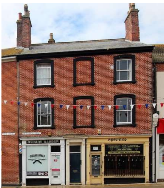
Nos.1-3 Saint Peter's Street
