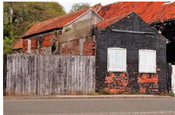
Detached store range to the south of No.329, Whapload Road
