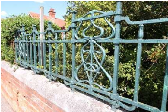
Boundary Wall and railings Nos.22-28 (even) Corton Road
