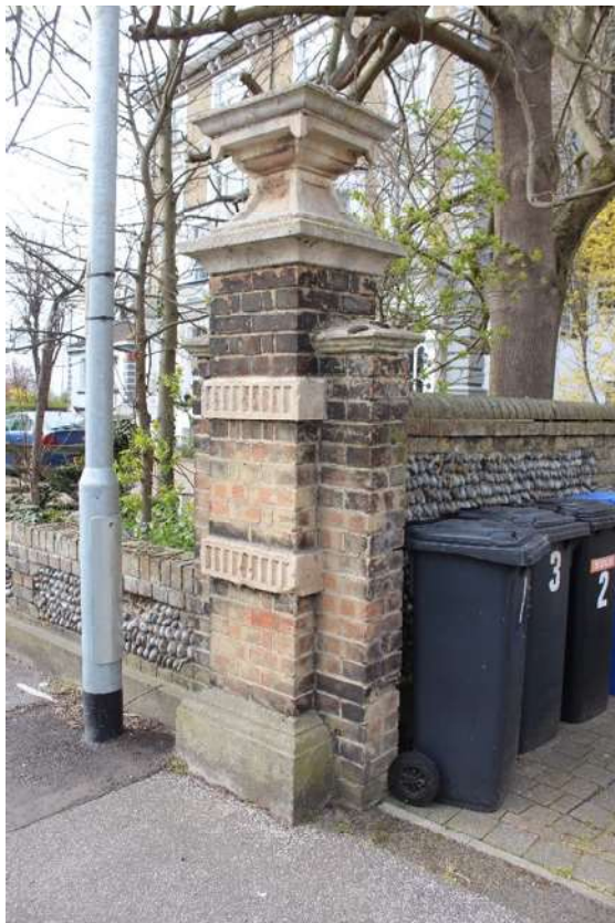
Gate pier, Wedgewood Court, North Parade
