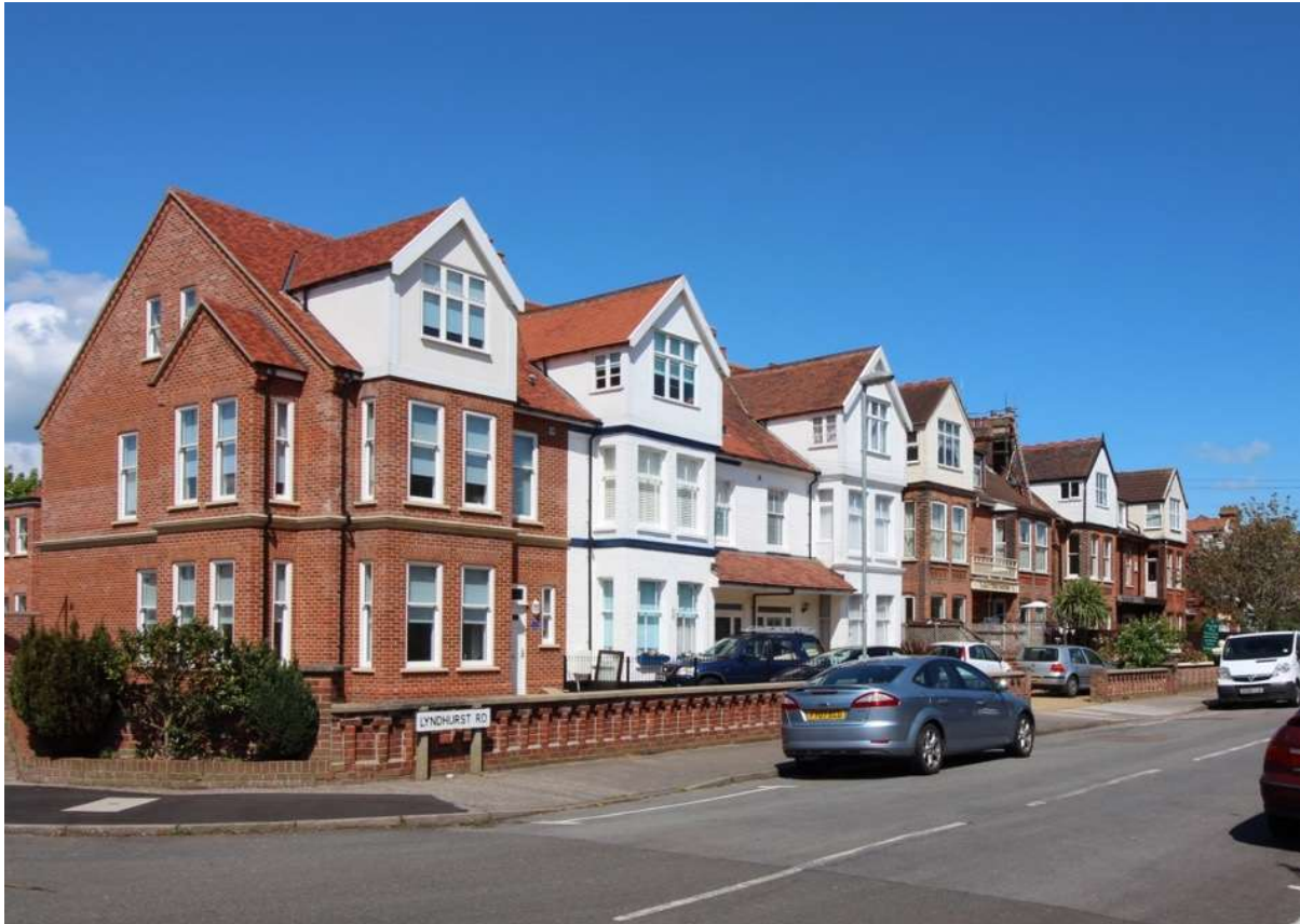
C2015 development at the corner of Lyndhurst Road and Corton Road, on the site of the fire damaged former Sunrise Inn.
