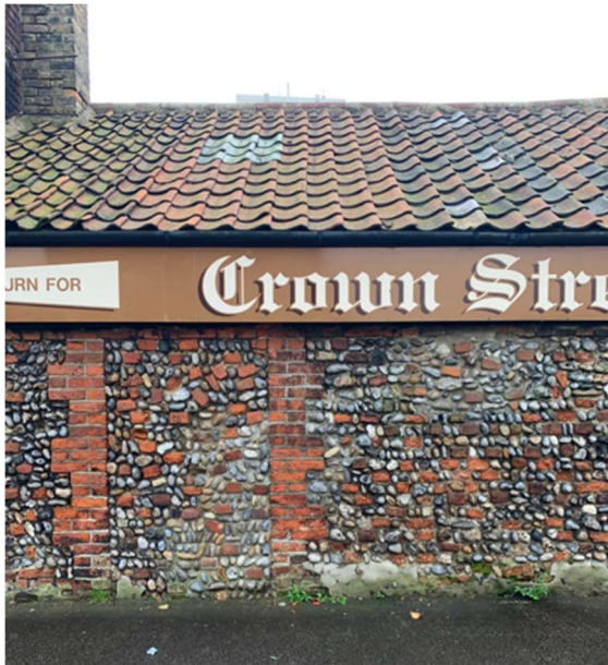
Brick and Cobble Wall to Crown Street Motors, Dove Street
