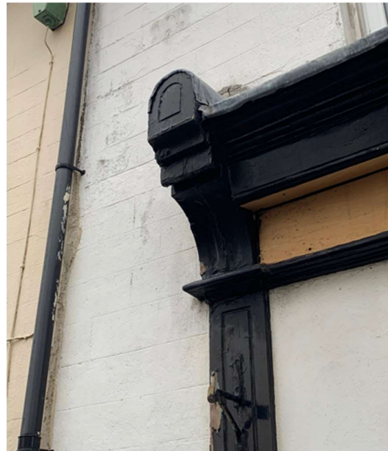
Detail of shop front to No.50, Crown Street West
