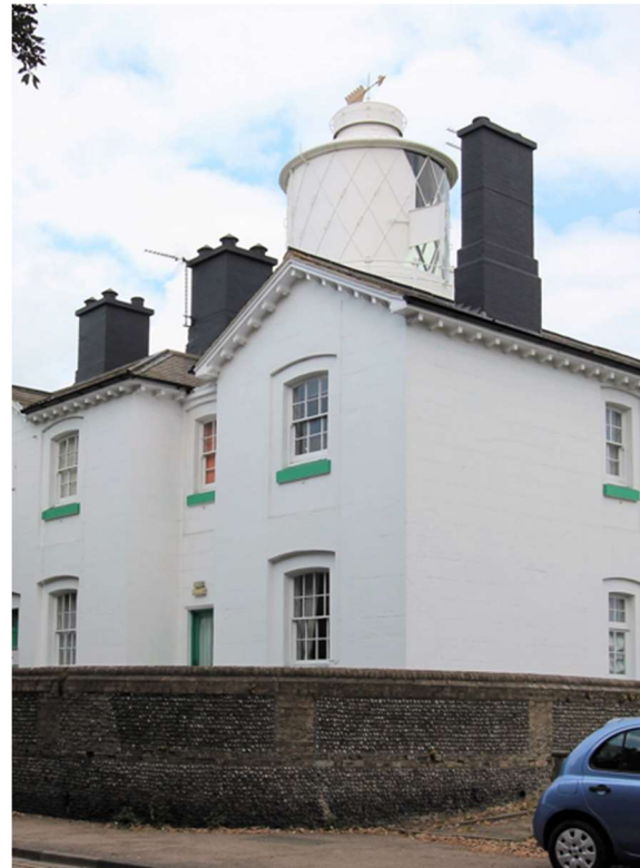
Rendered elevations with ashlar marking
