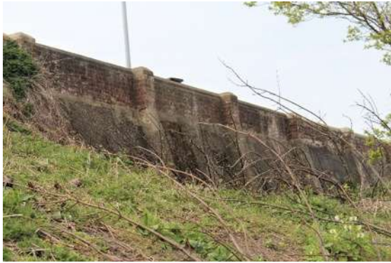
Retaining Wall and steps on the eastern side of Gunton Cliff
