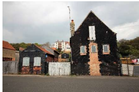
No.329 Whapload Road in 2018 with Arnold's House beyond.
