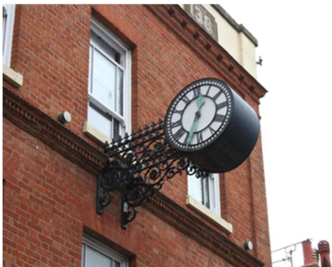
Projecting clock and bracket at No.138 High Street
