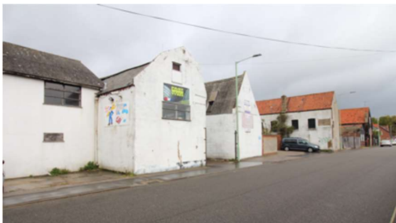
Painted brick and painted render elevations, and a variety of roof covering types
