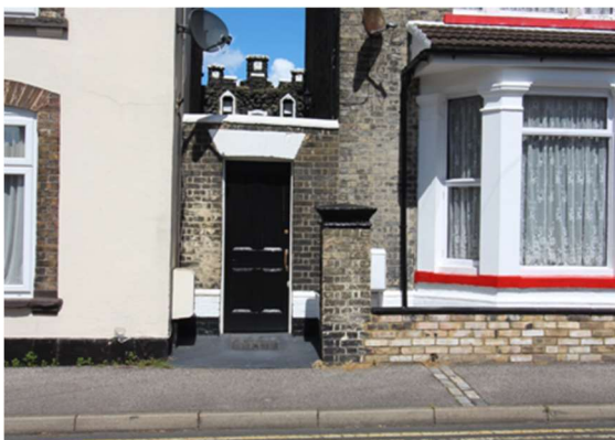
Detail of gate and structure behind, between no's 38a and 40, Crown Street West
