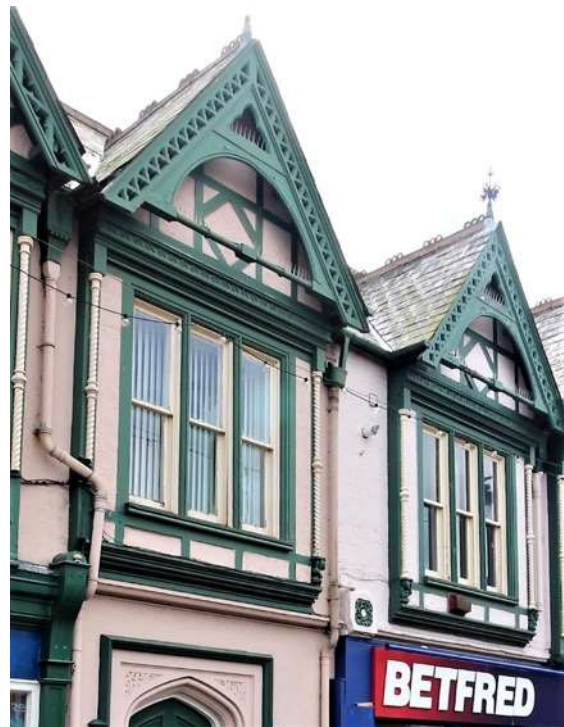
Detail of the façade to No.90
