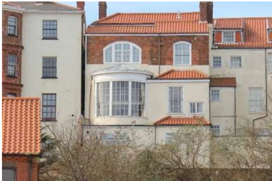
Eastern elevation of No.3 High Street
