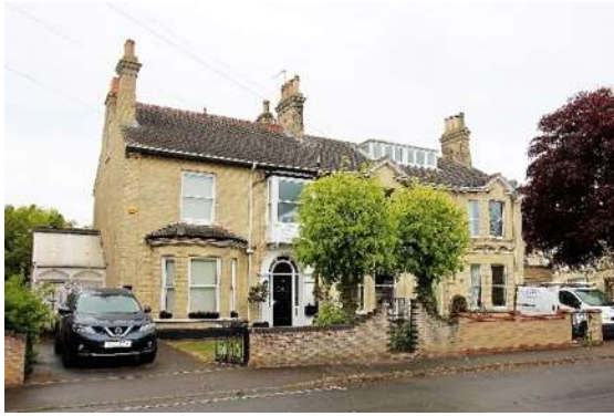
Nos.107 & 109 Park Road
