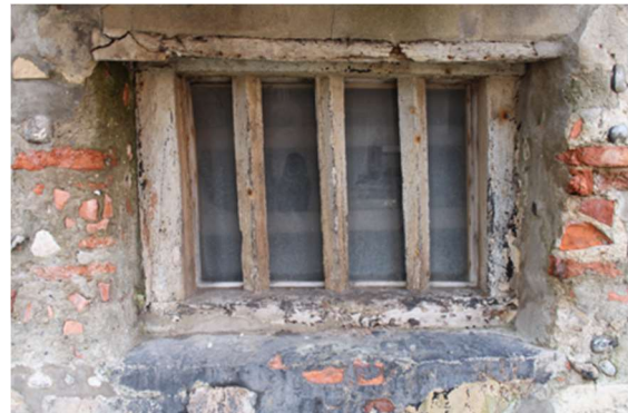
Detail of diamond set timber window or ventilator
