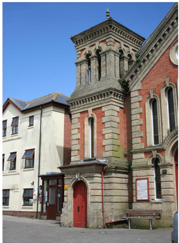
Red brick elevations with white brick dressings
