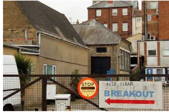
Northern elevation of Lowestoft Amateur Boxing Club
