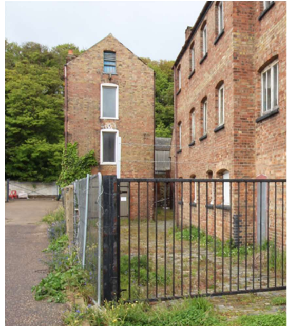
No. 311 Whapload Road, prior to commencement of conversion scheme.
