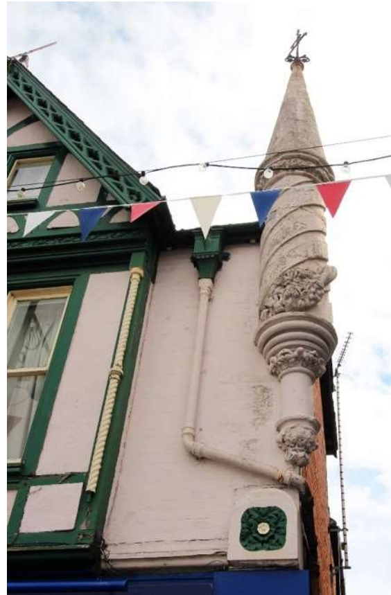
Detail of tourelle No.91 High Street
