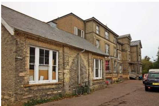
Abigail Court, southern elevation
