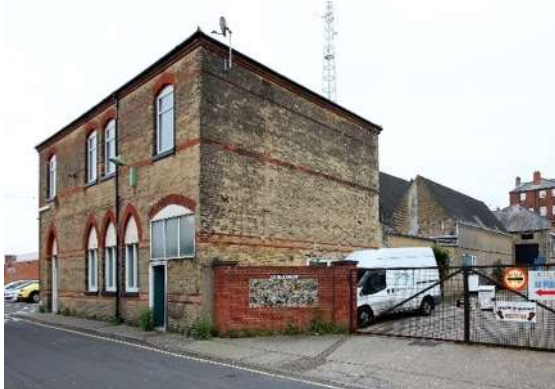
The Northern elevation of Christ Church Hall
