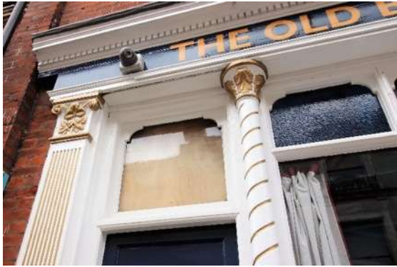
Detail of fascia, The Old Blue Anchor
