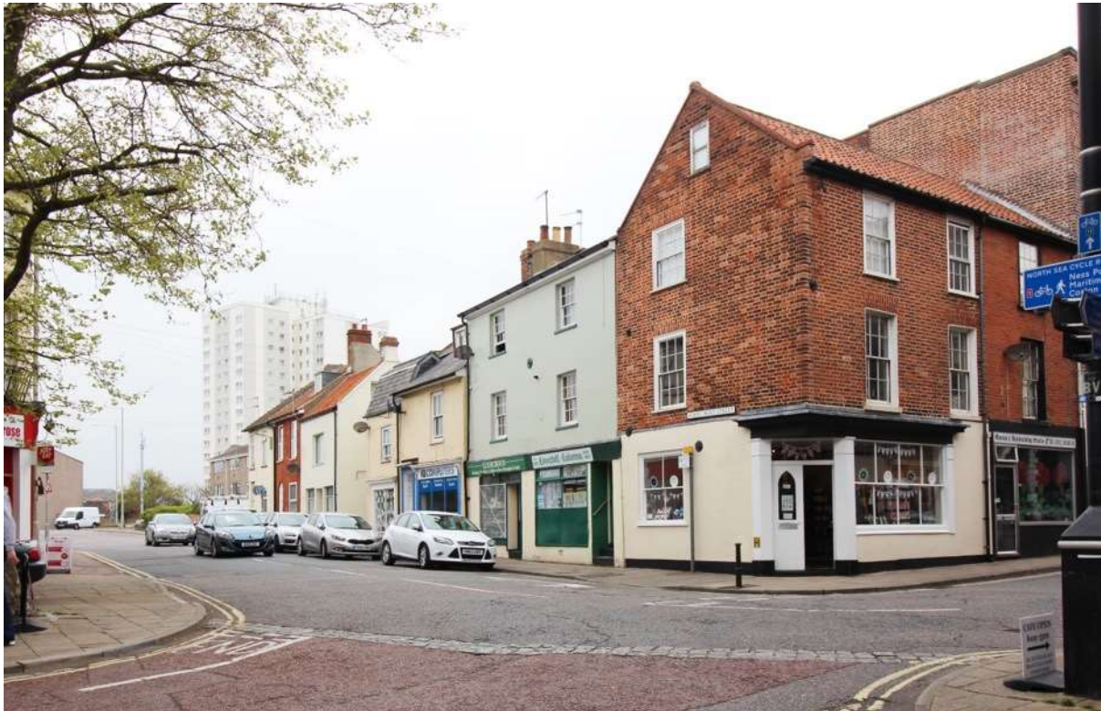
The fifteen storey St Peter's Court of 1967 dominates westerly views from the corner of High Street and Dukes Head Street
