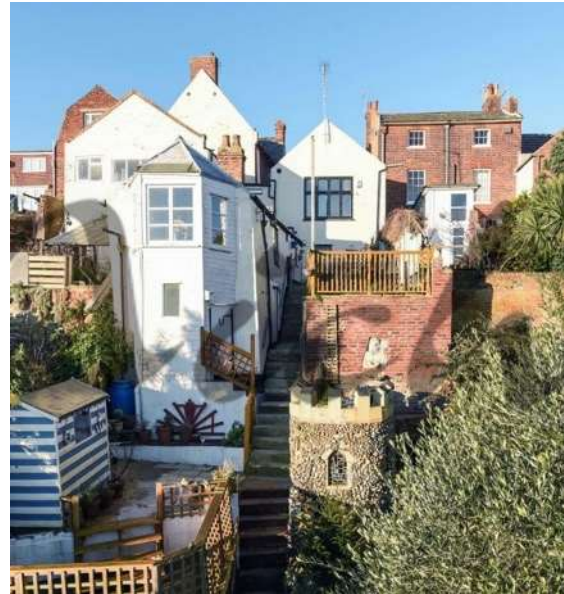
The rear of No.35 High Street
