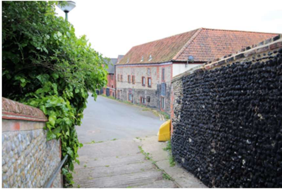
Cobble walls and red clay pan tile roof covering
