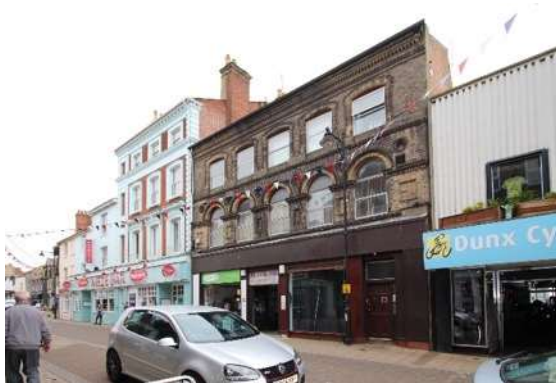
Poor quality shop fronts detract from the character of some High Street buildings, whilst the cladding added to No.100 (right) has badly disfigured its c1800 façade.
