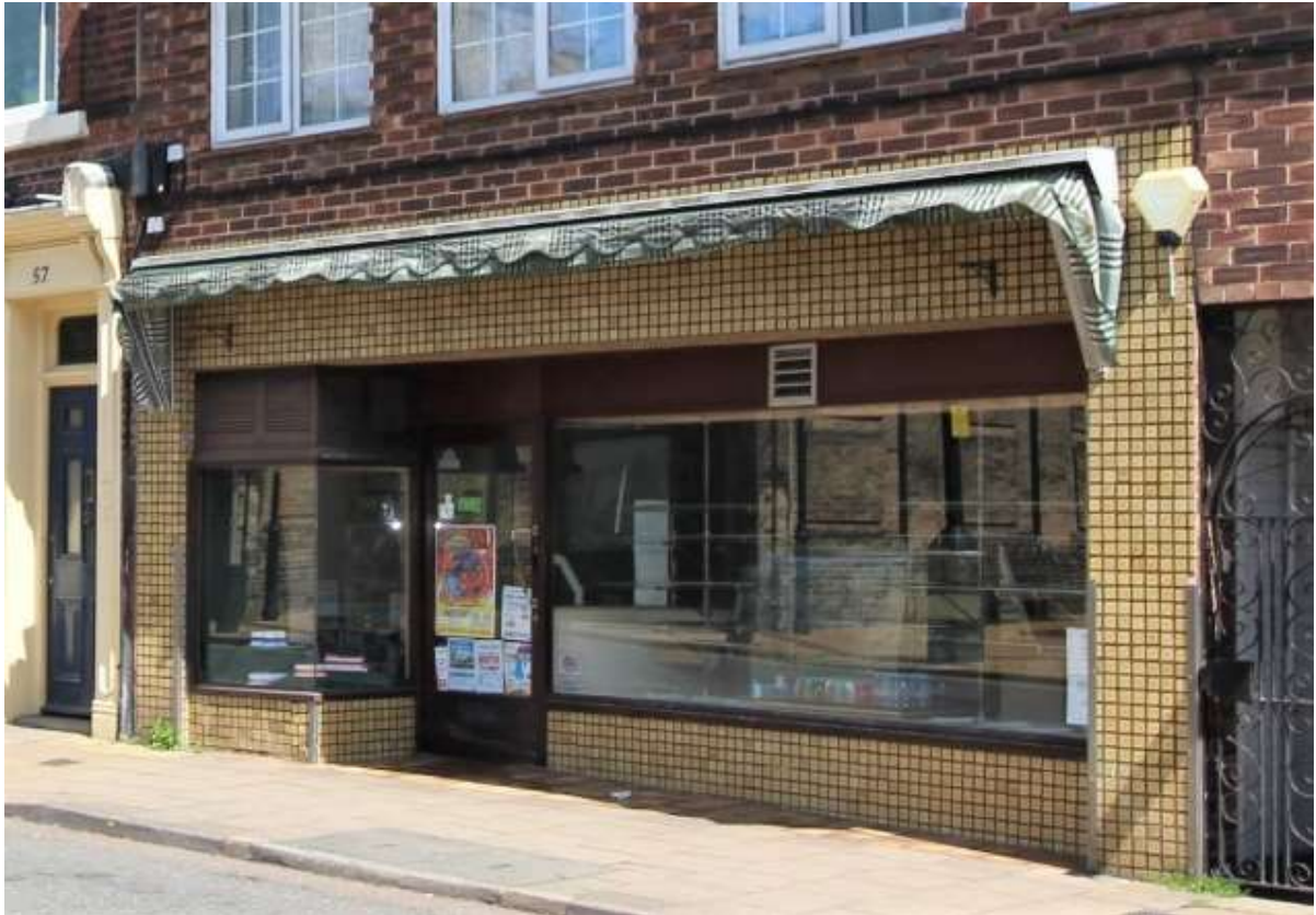
No.58 High Street retains a tiled bakery fascia and original display window of c1960. Historic England have emphasized the quality of its design and its remarkably intact state.
