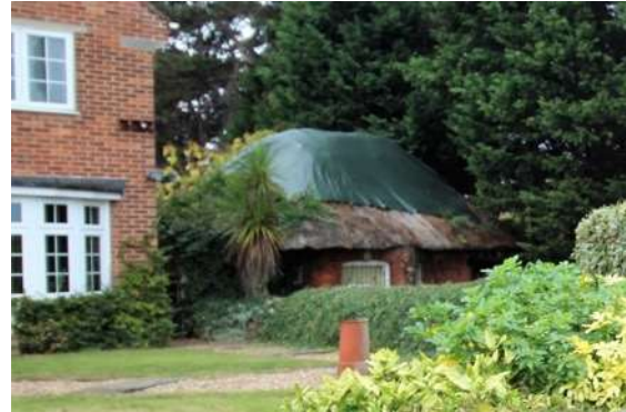
Garden Building at The Bleach, Heather Road
