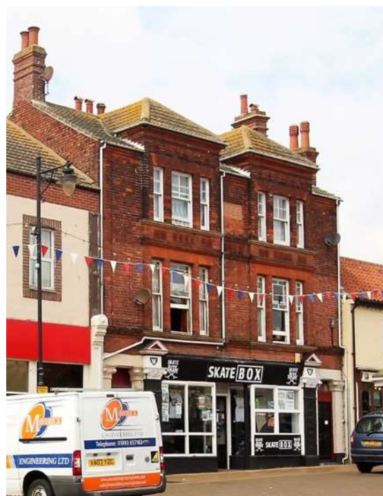
Nos.9 & 11 Saint Peter's Street
