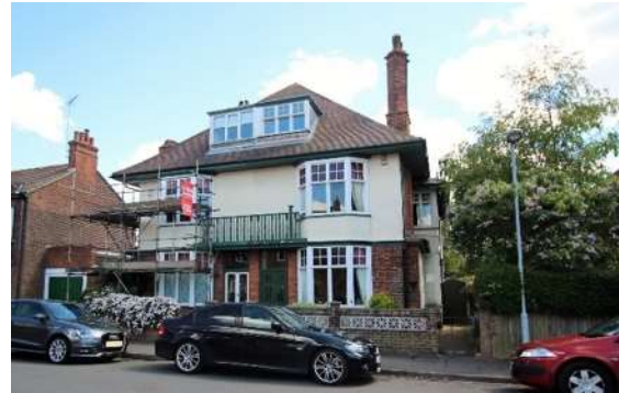
Park House and Park Side, Station Road
