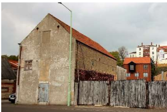
Eastern and northern elevations of No.325
