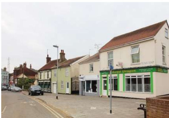
Surviving buildings at the southern end of St Peter's Street
