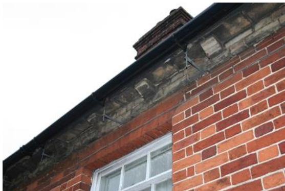
Gauged brick head and oblong panes of glass to windows, and unusual corbelled white brick eaves course detailing
