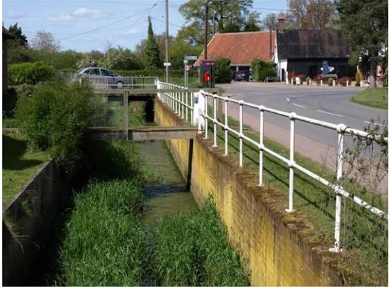
The channel through which the stream flows in this northern stretch of Pouy Street has been 'improved'. Cleared of much of the vegetation, a harsh brick retaining wall has been constructed, topped with a galvanised, tubular, metal balustrade.
