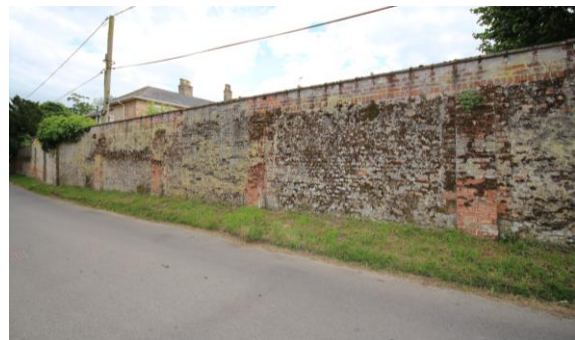
Flint and rubble incorporated into boundary walls
