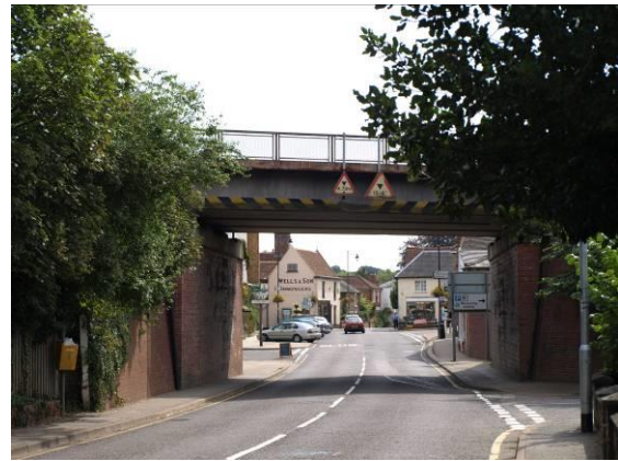
North entrance, looking south
