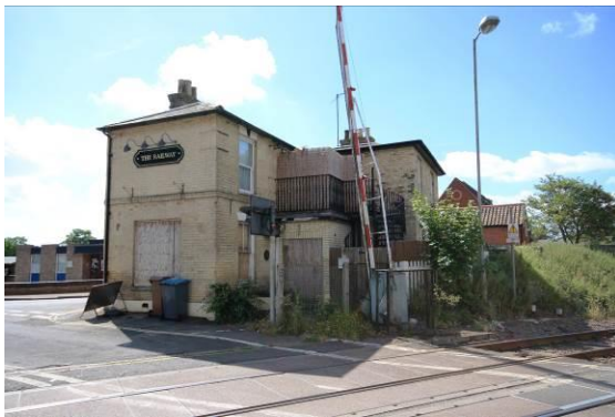
The Railway Public House, north-west elevation
