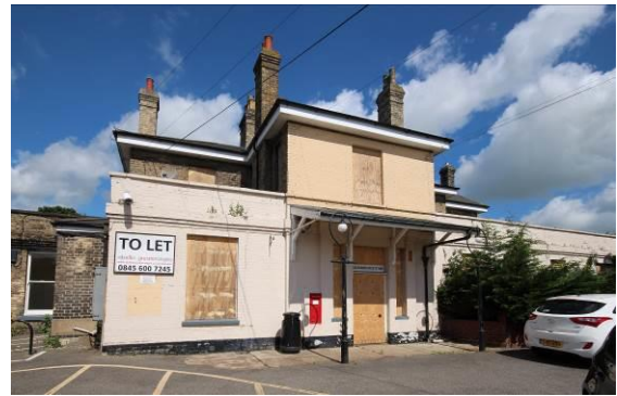
The Railway Station, south-east elevation
