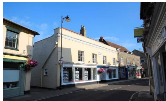
Re-fronting of an earlier structure, High Street
