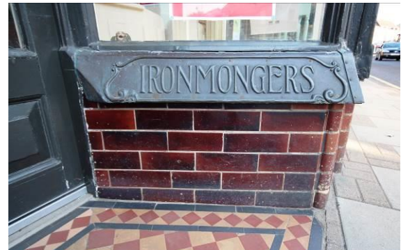
Detail of shop front, 46 High Street
