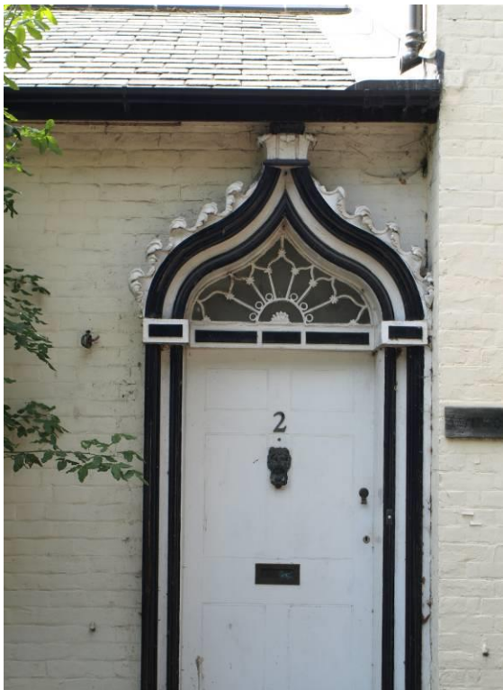
Painted brick, slate and an exceptional 'Gothick' doorcase
