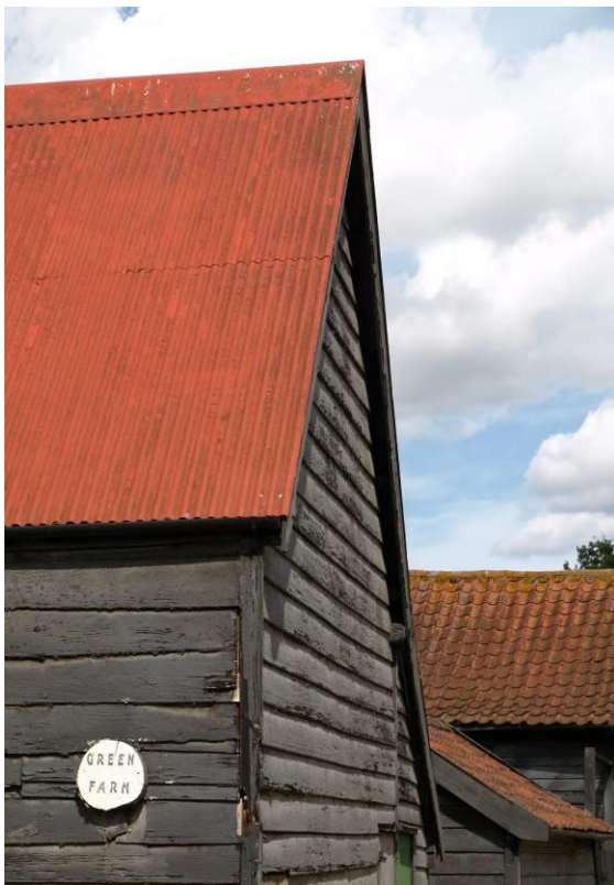
Weather-boarding and Corrugated Iron
