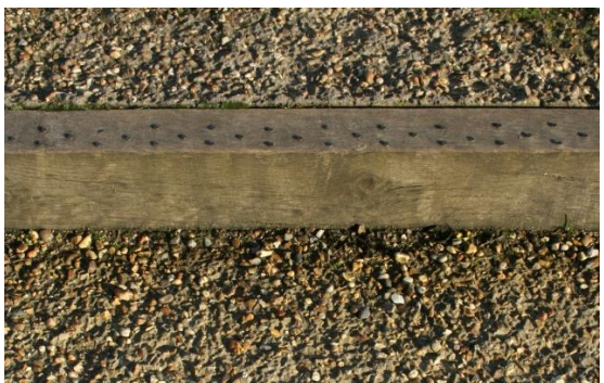
45) Timber nosing to steps with nail head detailing
