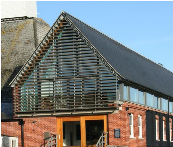
Slatted timber screen to upper section of gable end
