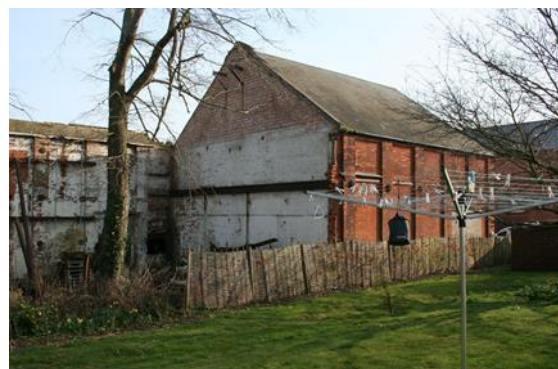
Southern elevation of south east range from the garden of Snape Bridge House showing scarring from the demolished section
