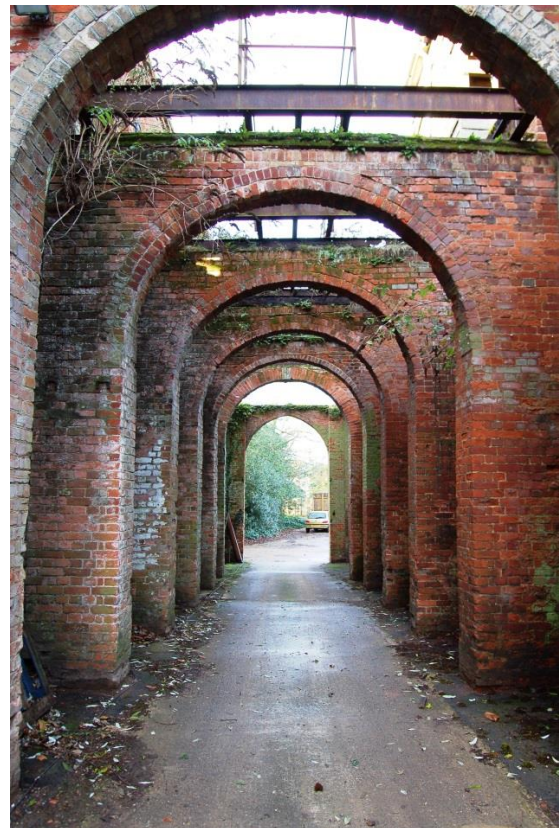
Brick relieving arches over passage way to the north of the warehouse dating from 1874.
