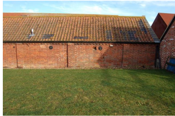
20) Brick dentil eaves decoration to former stable
