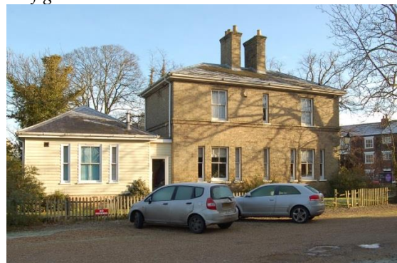
24) Gauged brick lintels and plate glass sash windows
