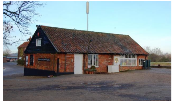
Gable end timber cladding to building 18
