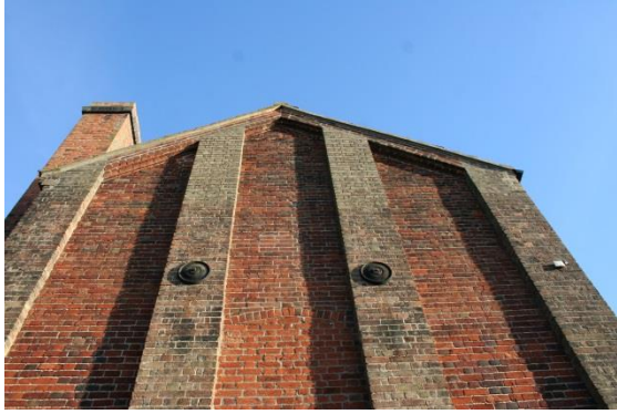
3) Red brickwork with gault brick dressings
