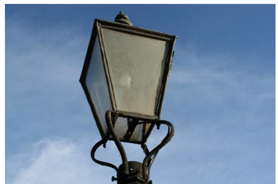
38) Glass lantern to converted gas lamp
