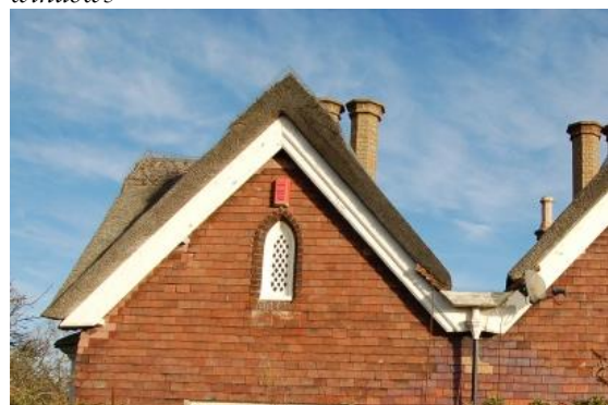
26) Gothic arch heads to windows with lattice glazing bars.
