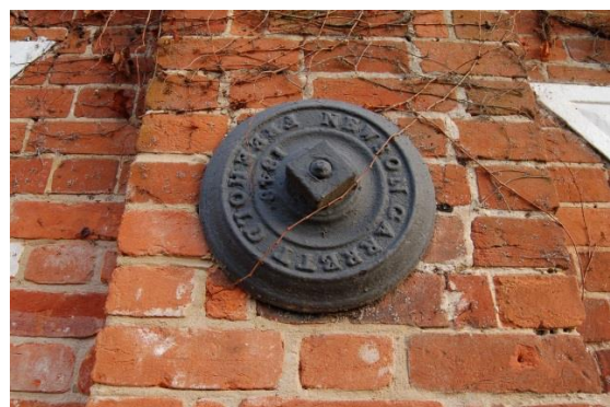
18) Cast iron pattress plates
