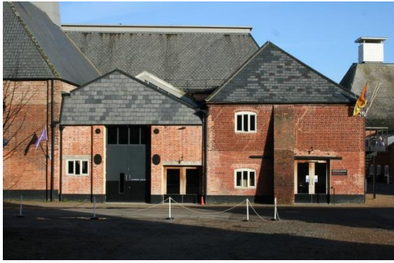
9) Slate roof coverings
