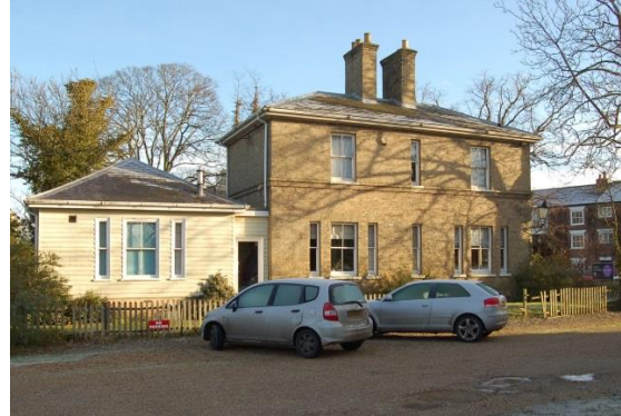
4) Gault brickwork and painted timber cladding
