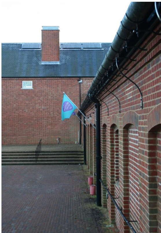
1) Red clay brickwork, of varying types and age
