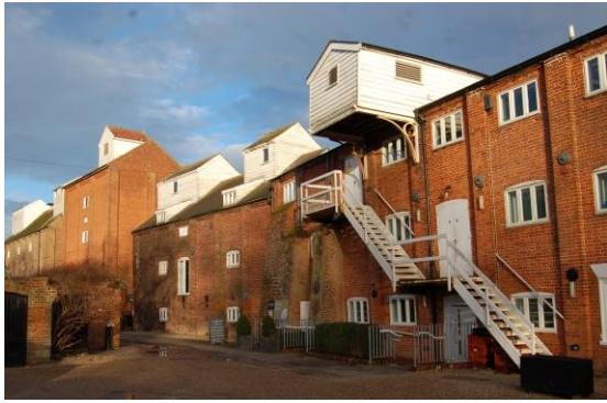
11) Projecting lucams and external stairs
