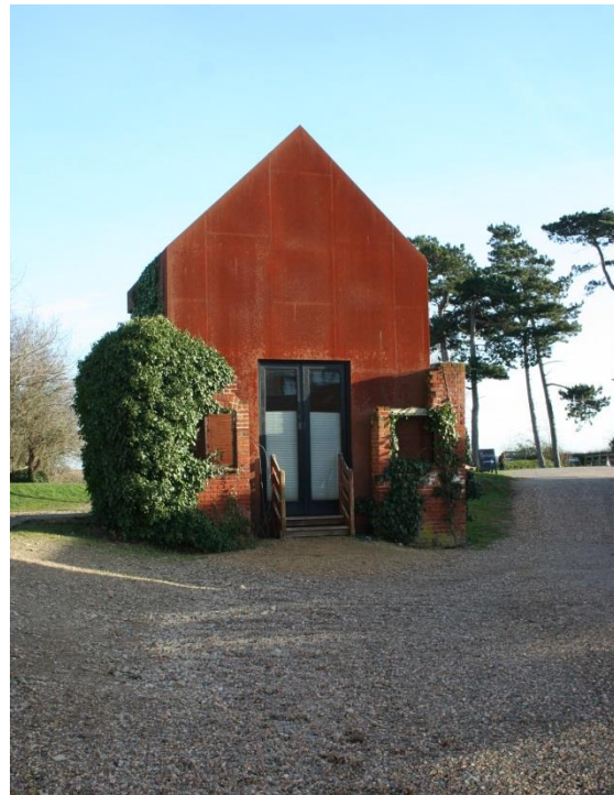
6) Corten steel construction
