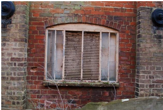
21) Shallow brick arch window heads and simple vertically divided windows
