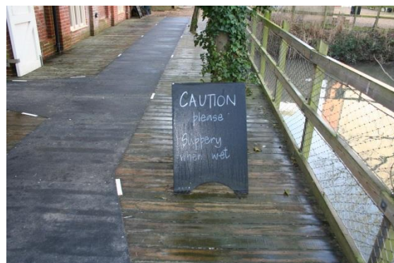
44) Timber decking with anti-slip felt
