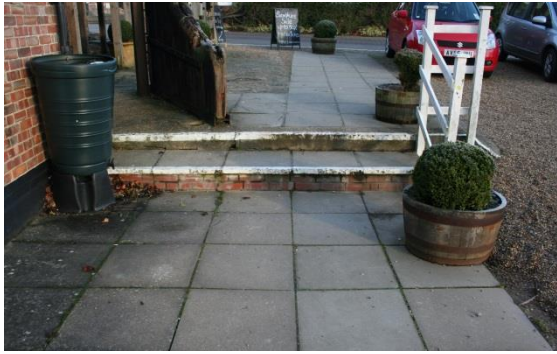
47) Concrete paving slabs to paths and steps
