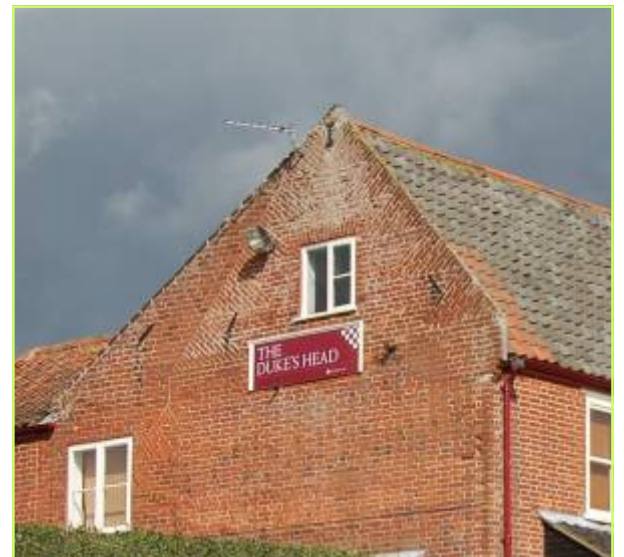
Fig 16, Gable end of the Duke's Head showing tumbled brickwork
