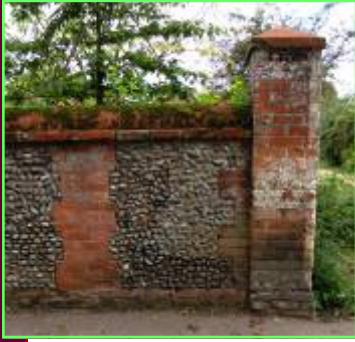
Fig 21, Cobble and brick garden wall, The Street c1860
