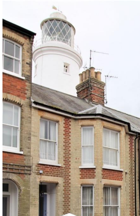
Chester Road: recently cleaned brick work.
