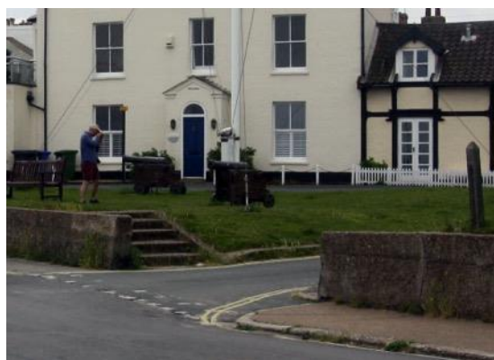
St James' Green: modern cement render (top) on earlier block wall and steps (below).
