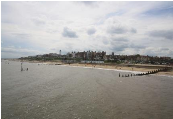
View of timber groynes, perpendicular to the coast and compartmentalising the beach to the south of the pier.
