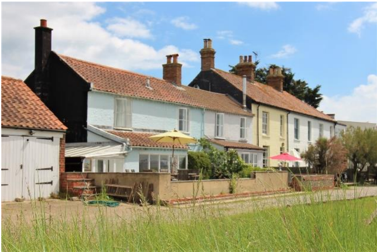
Blackshore Cottages from the southwest
