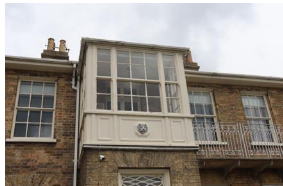
Timber square bay window.
