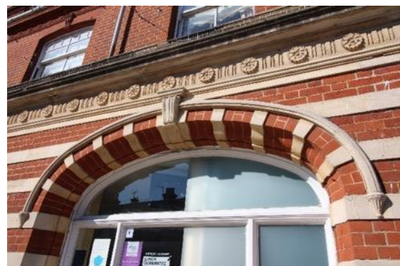
Detail of No.67 High Street.
