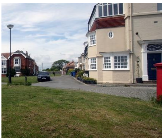
Granite Setts outside No. 2 Park Lane
