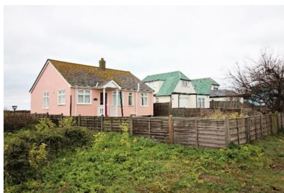
Nos.34-38 (even) Ferry Road
