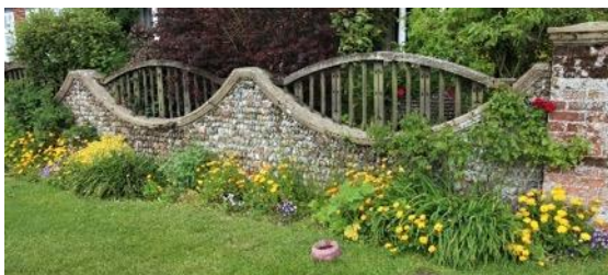
Cobble wall, stone caps and timber baluster screen to Commoners and Fairway Cottage, The Common
