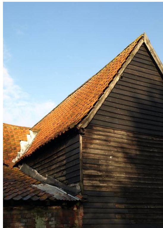
Weatherboarding and pan tile
