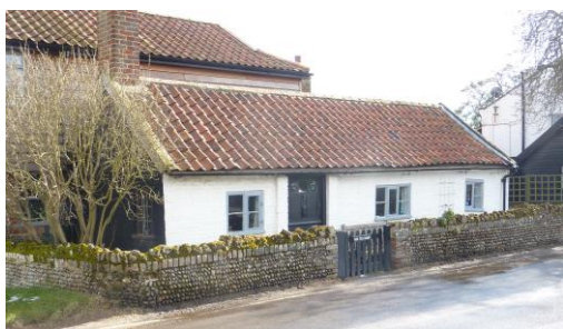
The Old Tea Room and boundary wall. Mid eighteenth century single storey front range (used during twentieth century as Tea Rooms) with two storey rear structure of uncertain date. Fronting the street is a cobble boundary wall with brick soldier course capping.
