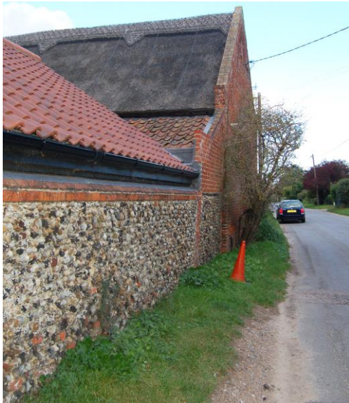
Wall in front of The Stables. Early to mid nineteenth century cobble, brick, clinker and knapped flint wall, with gault brick capping. Substantially complete, with little evidence of repair or rebuilding.
