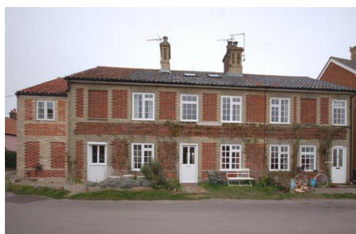
Lorne Cottages, 1, 2 and 3. Dated 1873. Red brick elevations with stone and gault brick dressings. Predominantly black glazed pan tile roof covering. Two red brick stacks located to the party walls, with gault
