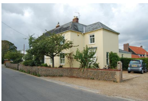
Manor Lodge, Manor House and boundary wall. Originally 'Manor Farm', early nineteenth century two storey rendered pair of cottages. Steeply pitched slate roof, with dentil eaves brick detail. Both cottages have additions to end gables. Also included is the cobble boundary wall, of predominantly early twentieth century date, with sections of later work and rebuilding.
