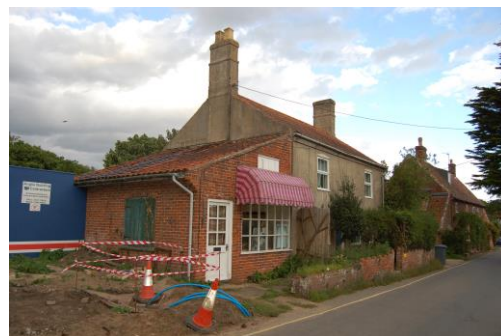
Alexandra Cottage, attached shop premises and boundary wall. Early to mid nineteenth century two storey detached brick cottage, now rendered, with attached red brick lean-to shop addition, of mid nineteenth century date, added to the west side. Crenellated early twentieth century boundary wall. Property forms key part of setting of neighbouring grade II listed property.
