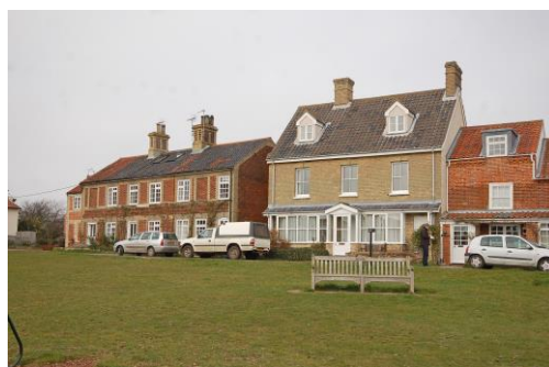
Dunwich View. Mid to late nineteenth century, three bay wide, two storey detached property with gault brick street elevation and red brick return elevations. Black pan tiled roof with two twentieth century dormer windows. Rendered east gable end. Four pane sash windows to the first floor, with projecting key stones. The ground floor openings have been replaced with a timber window arrangement that flanks the centrally located projecting porch.
