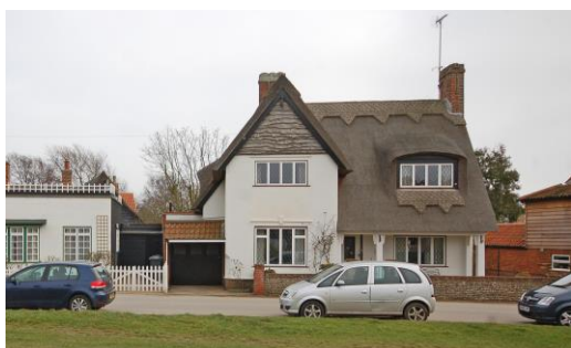
Greenways and boundary wall. Inter war detached dwelling with rendered elevations, thatched roof, eyebrow dormer and weather boarding to the upper section of the front elevation gable end. Ground and first floor windows have a projecting tile string course detail above openings, with the ground floor windows having key stone ornament. Good cobble boundary wall with brick capping and gate piers.
