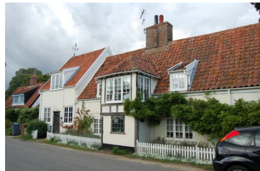
Westons, and boundary wall to east. One and a half storey dwelling with eighteenth century or earlier origins. 1785 date to east end gable may relate to re-casing. Two storeys projecting former entrance bay. Mid nineteenth century red brick wall with gothic detailing to gate opening.
