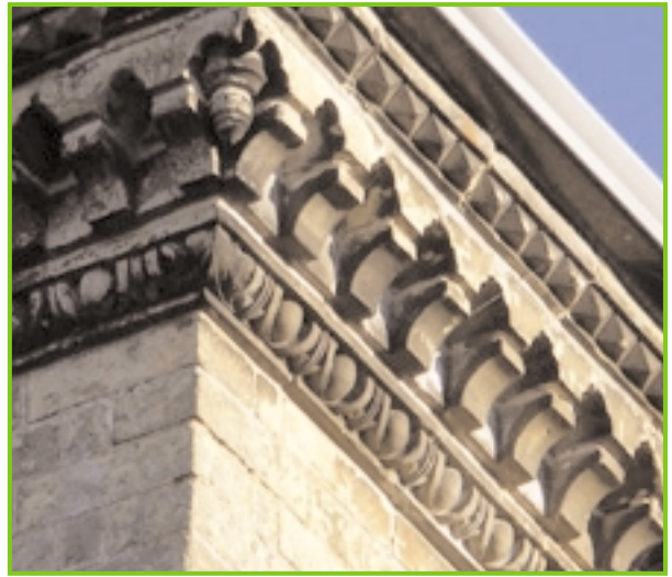
Moulded brick eaves detail, 16 High Street
