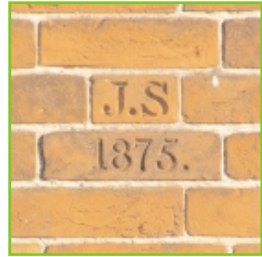
Initialed and dated red brickwork at no 13 Church St
