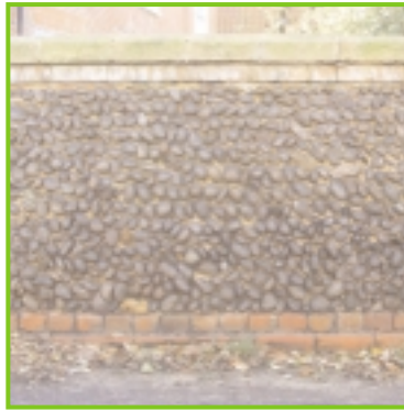
Cobble and red brick wall with white brick coping at no 2 Church St
