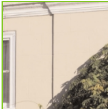
Ashlar detailing to 15 Church Street
