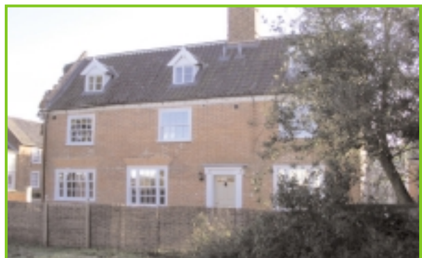
Little Priory, Church Street
