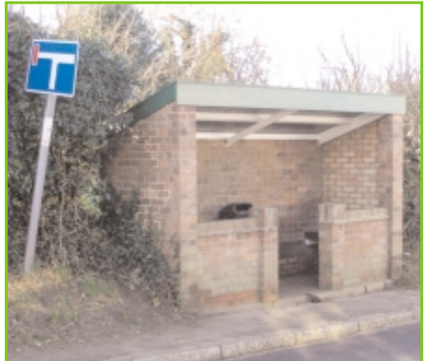
Bus shelter in Church Street
