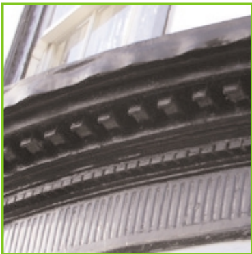
Detail of historic shopfront at 29 High St
