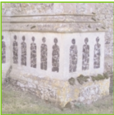
Knapped flint 'flushwork' detailing to church buttress
