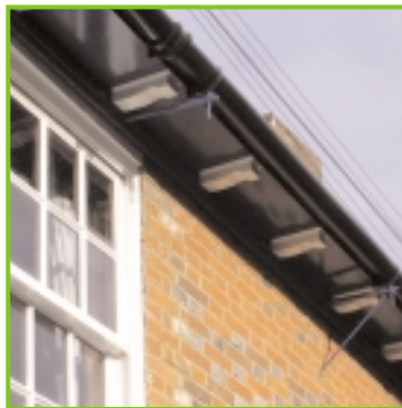
Decorative eaves brackets at no 13 High St
