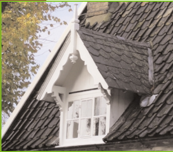
Historic 'pintle' window in fishscale-slatted dormer at no 1 High St
