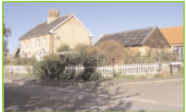
Outbuilding to south of 63 Church Street
