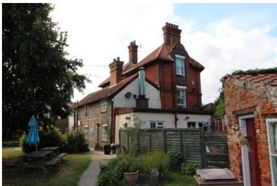
The White Horse Inn, Darsham Road. Rear south elevation showing the two distinct construction phases and one of the detached red brick outbuildings
