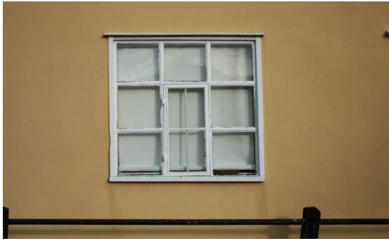
Figure 20: Timber casement window with opening metal casement hung on pintel hinges
