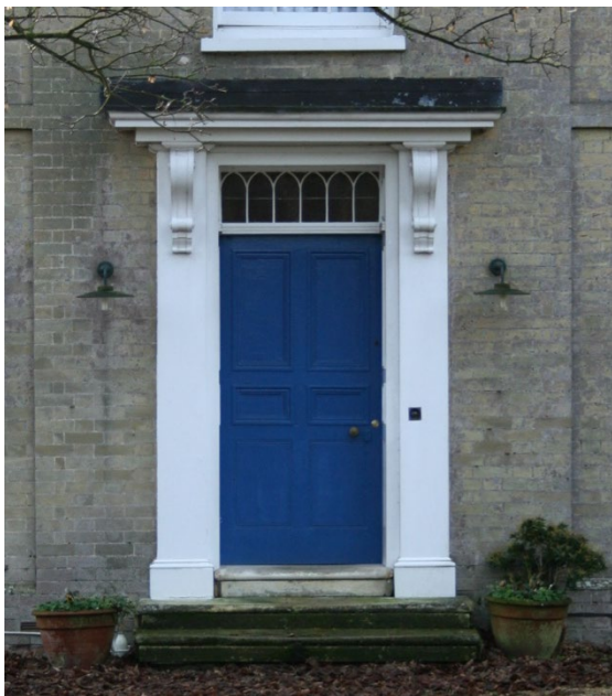
Figure 21: Timber doorcase, original door and overlight
