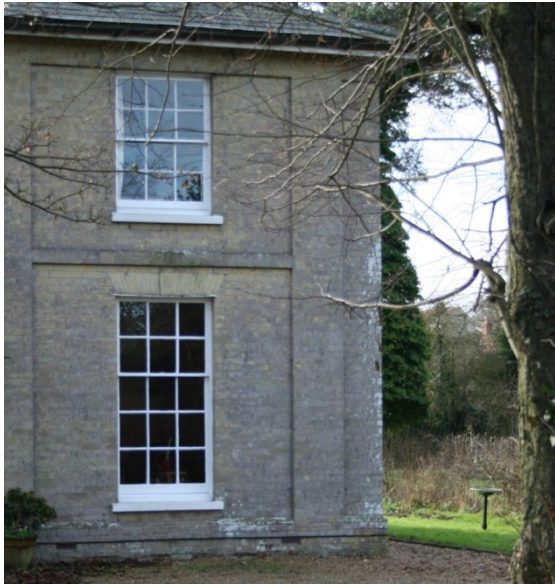
Figure 16: Gault brick and brickwork detailing
