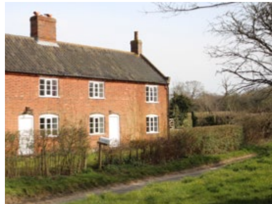
Figure 15: Good quality red brick cottages with black glazed pan tile roof covering and prominent chimney stacks
