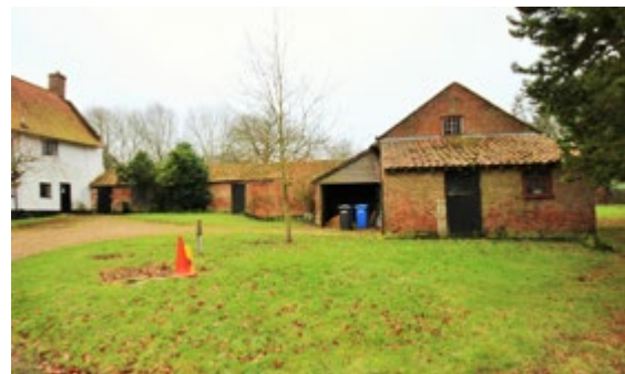
Figure 29: Attached outbuilding range and cart store, Whitehouse Farm, Mill Road
