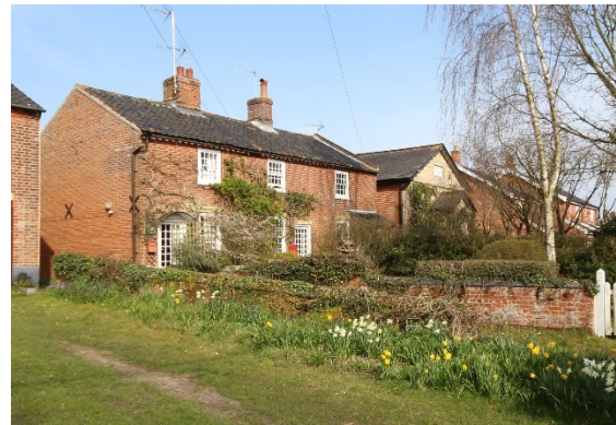
Figure 32: No's 2 to 4 (cons), The Street
