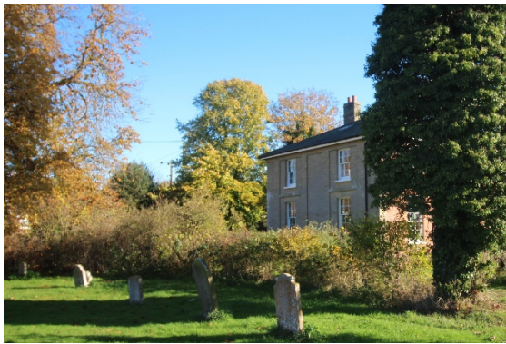
Figure 44: The Old Vicarage west elevation, seen from the churchyard
