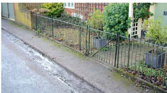
Figure 22: Retained iron railings and gate
