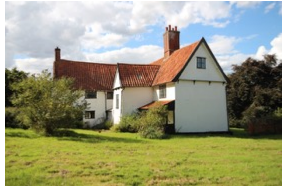
Figure 28: Whitehouse Farm, Mill Road, south east elevation
