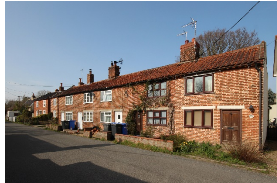
Figure 35: No's 13 to 17 (cons), The Street
