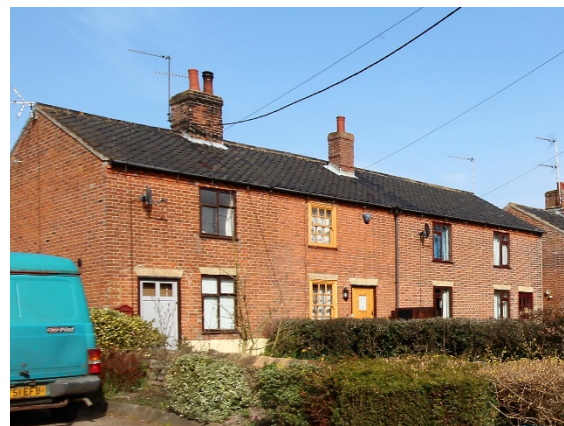
Figure 33: No's 5 to 7 (cons), The Street
