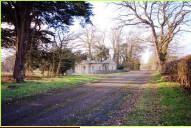
Fig 28, North Lodge Benacre Hall
