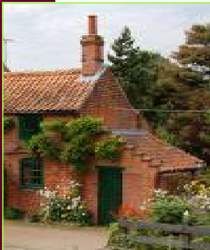
Fig 26. Detail of vernacular Architecture at No.15,High Street
