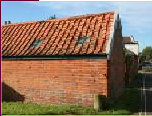
Fig 23. Example of local red clay Brickwork and roof tiles
