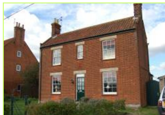
Fig 35, No.25 Mill Lane
