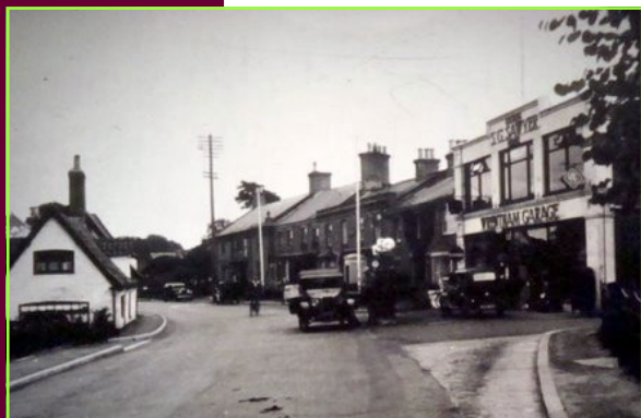
Fig 10. Historic View, c1920, showing Wrentham Garage (now Boggis Electrical)
