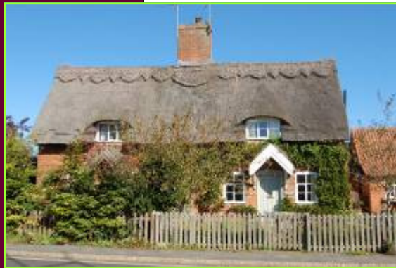
Fig 16. Grade II listed cottages at No's 4-6, Chapel Road
