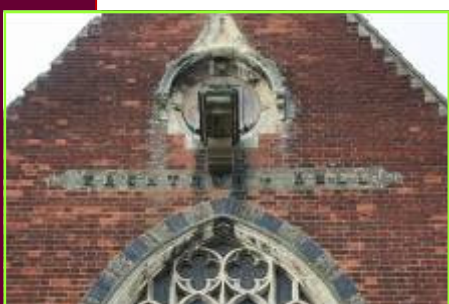
Fig 19. Detail of stone carving to the former Town Hall, High Street
