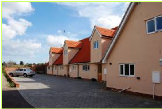
Fig. 12, Old Bank Mews which it is proposed to remove from the conservation area
