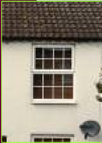
Fig 22. Example of replacement UPVC windows
