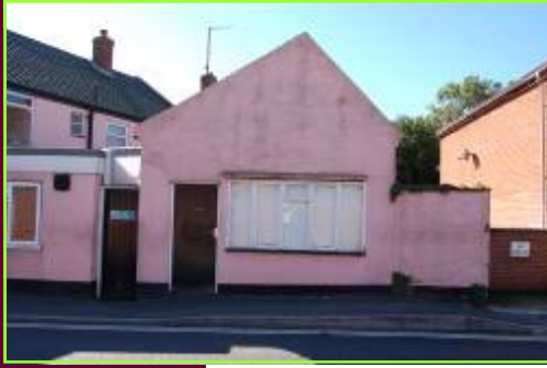
Fig 31. No.3, Chapel Road, outbuilding
