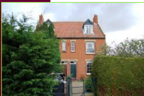
Fig 53. No's 2 to 4, Priory Road
