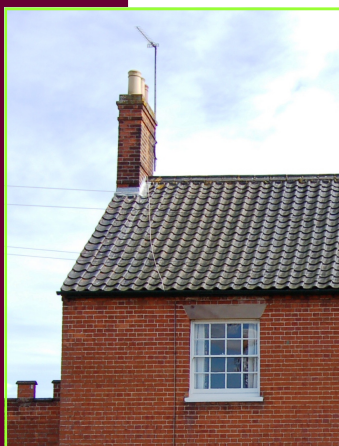
Fig 24. Example of sash window and Black glazed pan tiled roof
