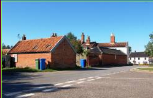
Fig 52. Outbuildings to the rear of No.1 Southwold Road, as seen from Mill Lane
