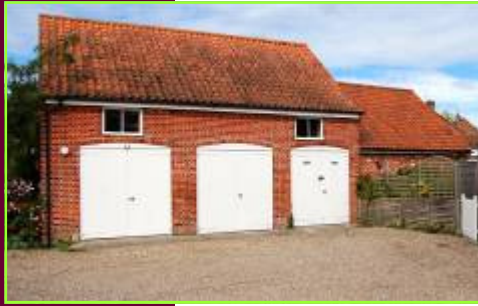
Fig 35. Former Cart Stores to the NW of Eagle Court
