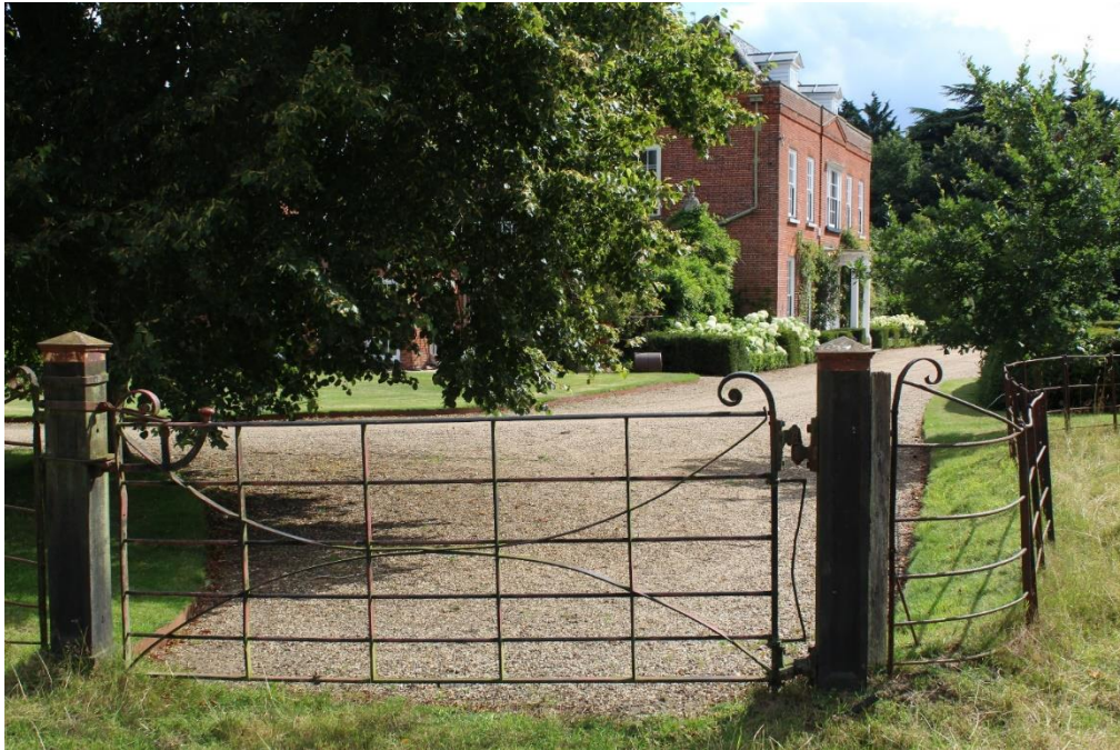
Figure 6 Historic gate and fencing with North Cove Hall and garden beyond
