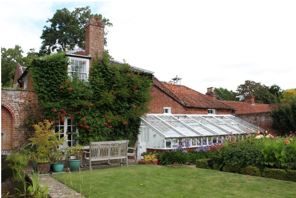
Figure 19 Gardener's cottage which flanks the walled garden, and view towards the greenhouse which displays the curved glass roof
