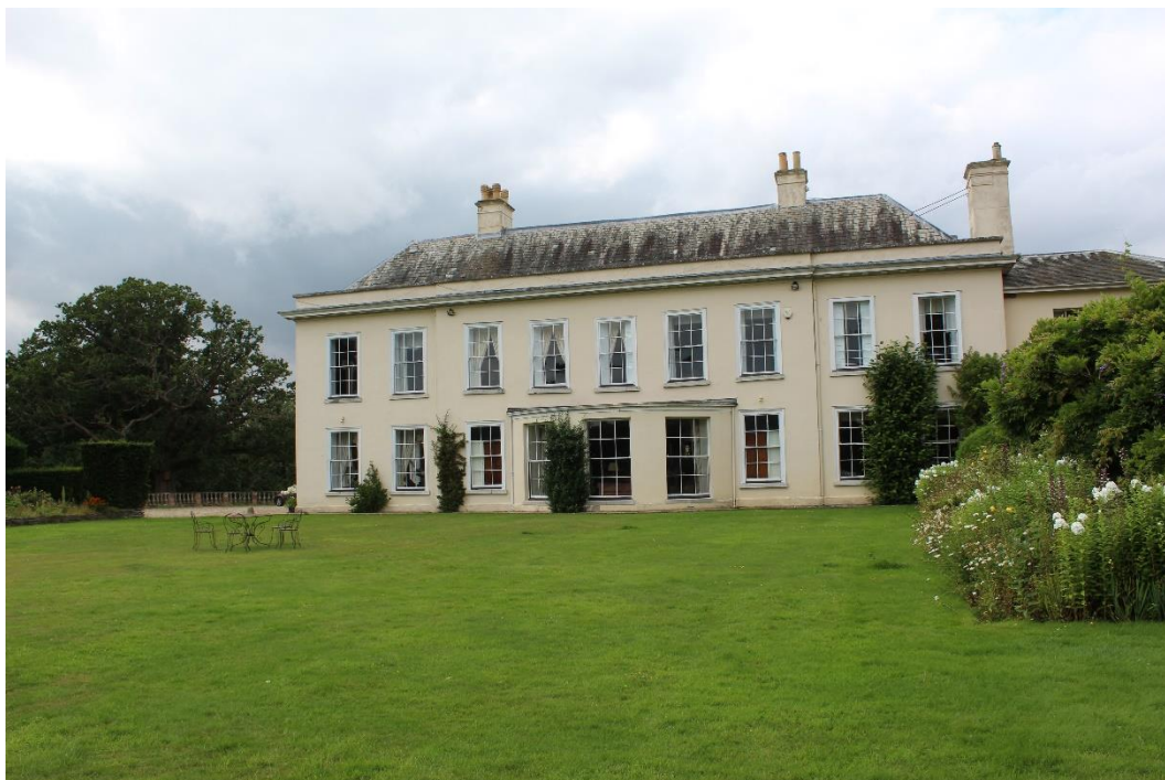
Figure 30 View of the hall from the garden to the east
