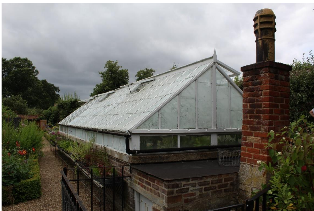
Figure 17 Greenhouse with boiler
