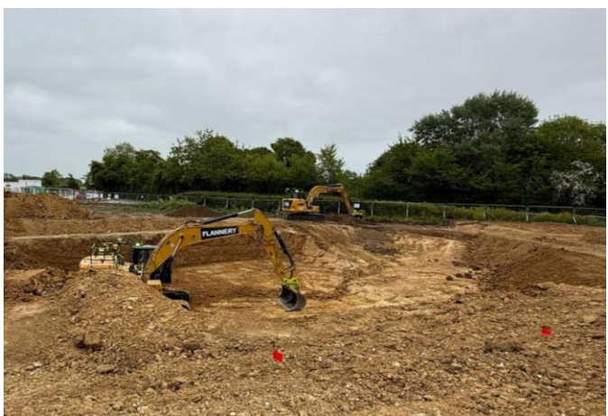
Attenuation Pond Construction
