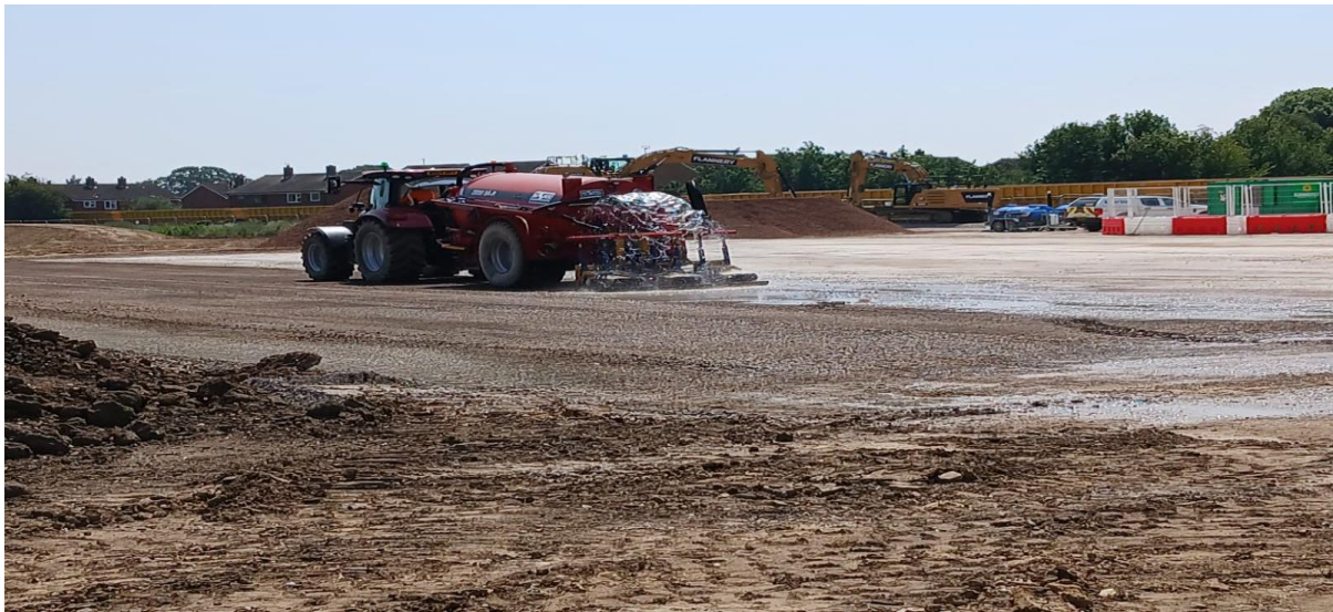
Soil Stabilisation (completed)
