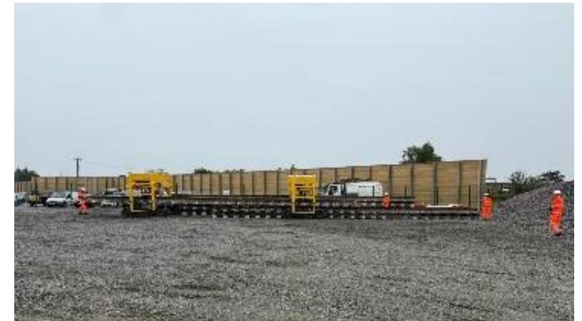
79 Nr Track Panels being stored in the ACA
