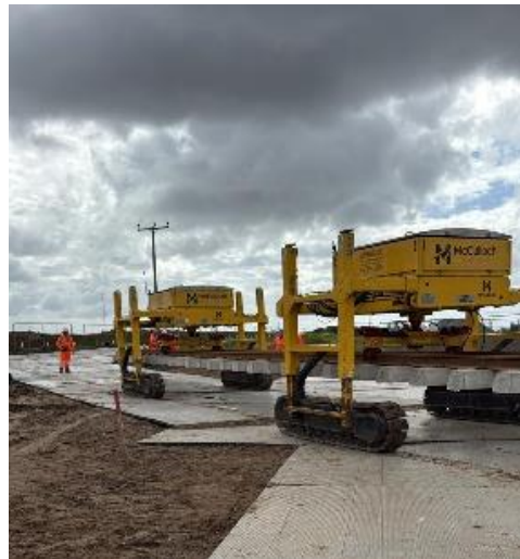
Plain line Track Panels Delivery
