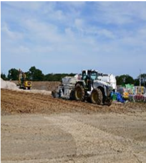
Soil Stabilisation (completed)
