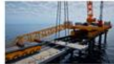
5. Precast concrete slab installation on the rear side using 300T crawler crane
