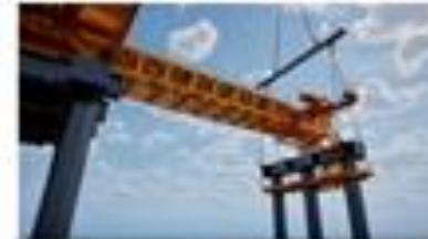
2. Capping beam installation on piles
