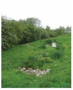
Figure 23.11 Balancing pond with marginal wetland treatment zone, Hopwood Park motorway services, M42, Worcestershire
