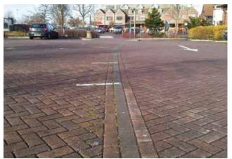
Figure 8.4 Lined permeable pavement constructed over a
