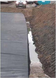
Figure 21.21 Flotation and movement caused by rainwater in excavation (courtesy EPG Limited)
