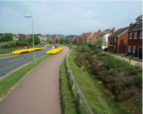
Figure 9.18 Swale set back from road, Elvetham Heath (courtesy Hydro International)
