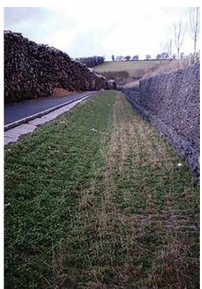
Figure 17.6 Swale with vertical side (courtesy EPG Limited)
