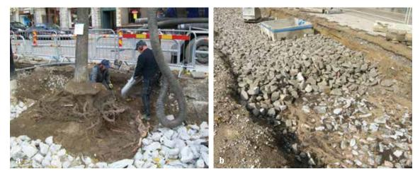
Figure 19.7 The use of structural growing media in retrofitting (a) and new-build (b) (courtesy Björn Embrén)
