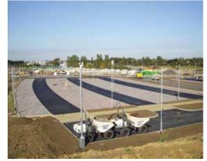
Figure 20.1 Park and ride scheme on the outskirts of Cambridge using concrete block permeable paving (courtesy EPG Limited)
