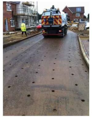
Figure 20.29 Layer of protective DBM over sub-base after coring and before laying concrete block permeable paving (courtesy Peterborough City Council)
