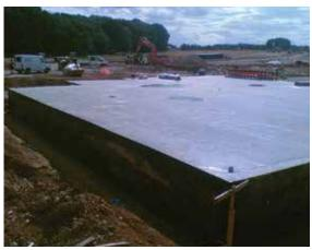
Figure 21.3 Frame covered by outer skin (geomembrane in this case) (courtesy EPG Limited)
