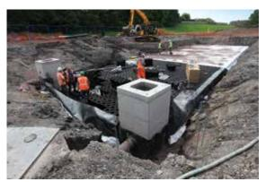
Figure 21.5 Man access chambers located within the structure (courtesy Aco Limited)
