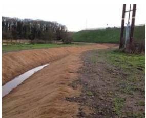
Figure 30.7 Example of coir matting for a swale (courtesy Stormwater Management)
