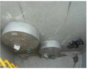
Figure 28.26 Two passive devices for multiple flow control (courtesy Hydro International)
