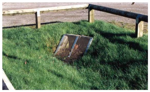
Figure 28.15 Example of screened orifice outfall with T-piece structure (courtesy Robert Bray Associates)
