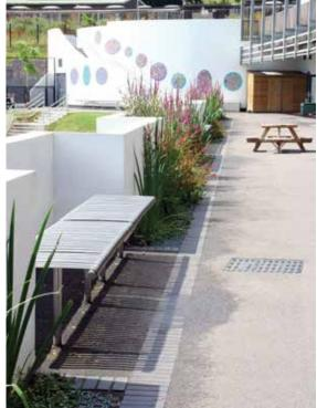
Figure 16.4 Filter drain with planting, Exwick, Devon (courtesy Robert Bray Associates)
