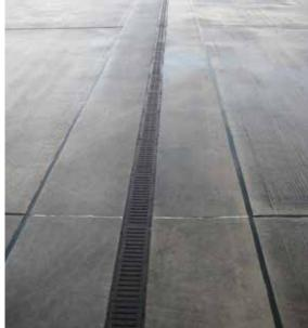
Figure 20.9 Macro pervious pavement in warehouse yard in north-west England with channel collection/ pollution trap and concrete pavement construction (courtesy EPG Limited)
