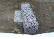
Figure 8.8b Check dam in a swale during construction, Lincoln (courtesy Lincolnshire County Council)
