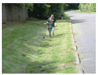
Figure 17.17 Grass cutting of roadside swale, Stirlingshire (courtesy Abertay University)
