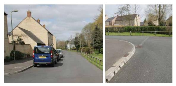
Figure 9.16 Kerb drains and channel connected to swale (courtesy EPG Limited)
