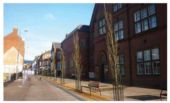
Figure 19.13 Linear tree pit, Leicester (courtesy Leicester City Council)
