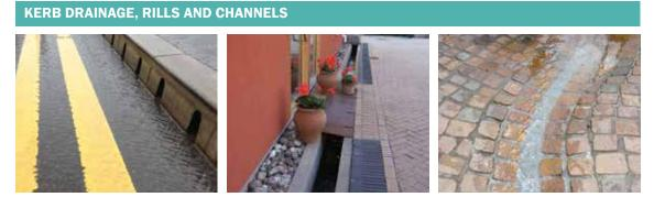
Figure 10.3 Kerb drainage, rills and channels (courtesy ACO, Illman Young)
