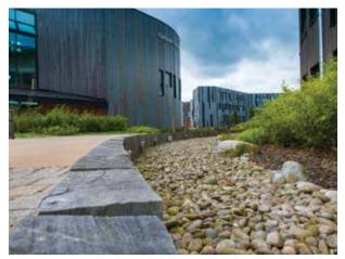
Figure 28.5 Timber sleeper edging with gaps, University of York (courtesy Arup/Giles Rocholl Photography)
