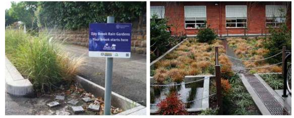
Figure 18.11 Example of a bioretention system with a simple sediment forebay, Nottingham (courtesy Environment Agency)
