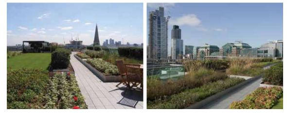
Figure 12.4 Examples of accessible green roof with intensive and extensive planting, Bishops Square, London
