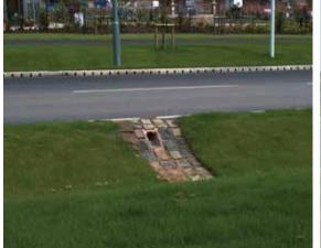
Figure 9.17 Outlet from kerb drain into swale (courtesy ACO Limited)
