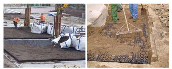
Figure 19.10 Geocellular systems for trees, showing filling of geocellular rafts with structural growing medium (courtesy Permavoid Limited and EPG Limited)
