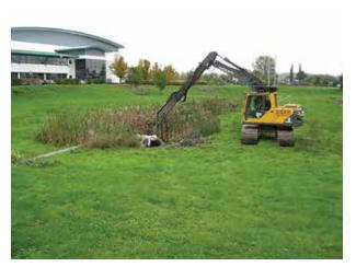
Figure 32.2 De-silting (courtesy Bedford Group of Drainage Boards)
