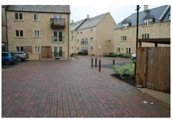
Figure 20.20 Concrete block permeable paving after a 50 mm rainfall event (courtesy EPG Limited)
