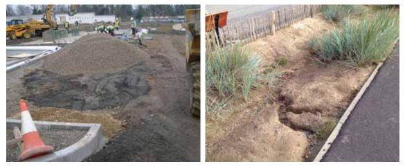
Figure 31.1 Inadvertent compaction of subgrade below pervious surface construction intended to infiltrate water to ground. Compaction will reduce the infiltration rate (courtesy EPG Limited)
