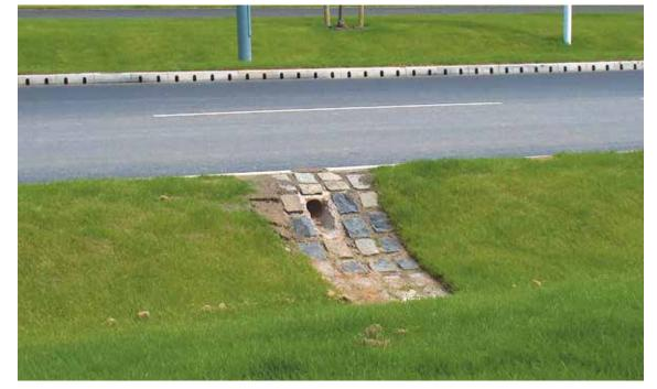
Figure 28.7 Kerb collection system being used to drain a carriageway in conjunction with a swale (courtesy ACO Limited)
