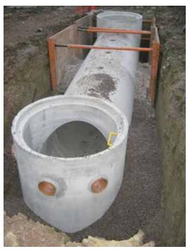
Figure 21.9 Direct access chamber into concrete pipe (courtesy British Precast)
