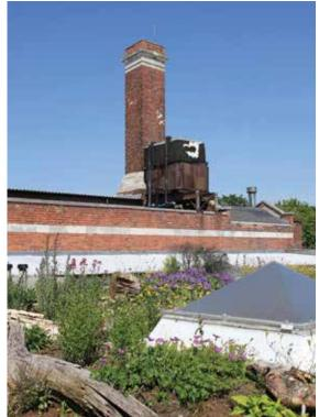
Figure 12.11 Biodiverse green roof, Unicorn Grocery, Manchester (courtesy Unicorn Grocery)
