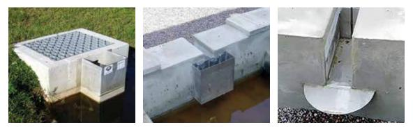
Figure 28.27 Examples of debris guards over low-flow outlet control structures (courtesy Robert Bray Associates)
