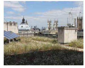
Green roof (courtesy Green Roof Consultancy) Figure 1.4 SuDS providing urban cooling
