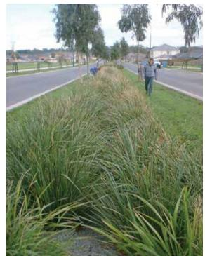
Figure 18.7 Bioretention swale (courtesy Derwent Estuary)
