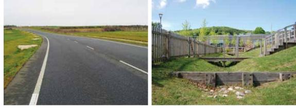
Figure 17.14 Roadside swale with granular check dams (courtesy Oxfordshire County Council)
