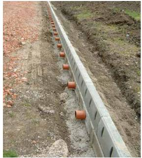
Figure 20.8 Macro pervious pavement under construction in the Midlands – kerb drain collector/ pollution trap with connectors before placing diffusers and permeable sub-base to left (courtesy Phil Tomlinson)
