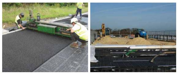
Figure 20.10 Construction of sports drainage and attenuation layer below school sports pitch in Hull (courtesy Phil Tomlinson)
