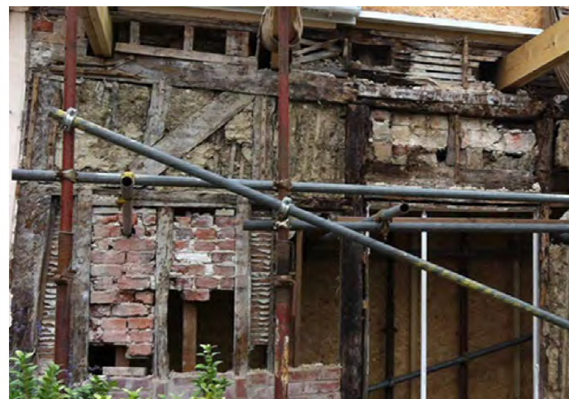
Repairs to a wattle and daub wall (note sections of brick used as a replacement on the ground floor) (The Agent's House, Easton). (Source - Roberts Molloy Associates)
