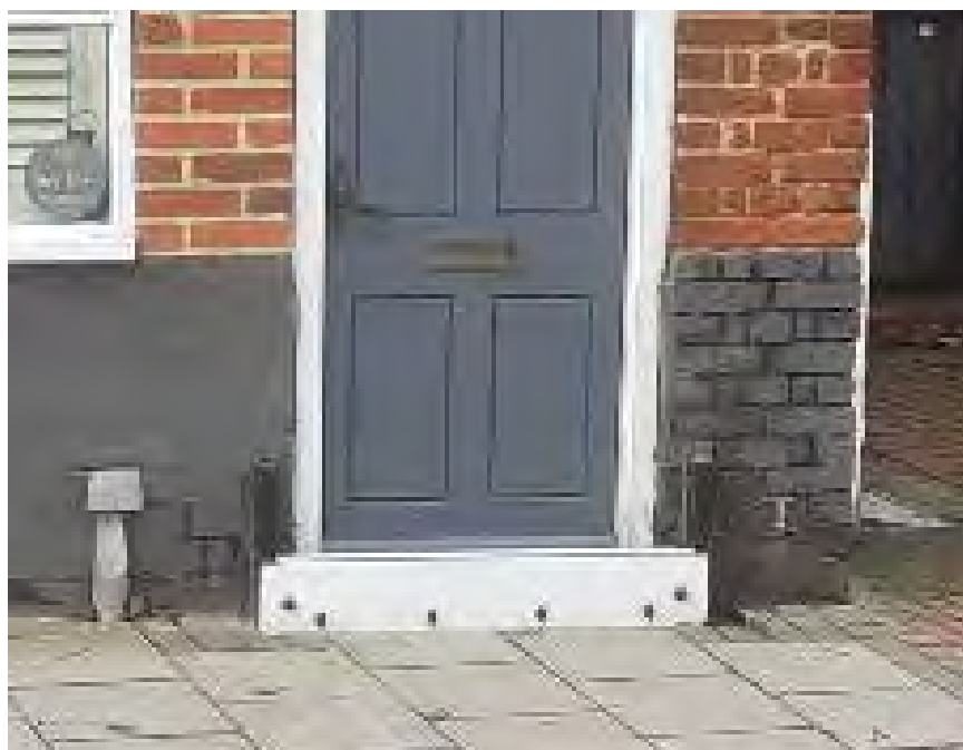
Flood barrier protecting the door of an historic building (Woodbridge)
