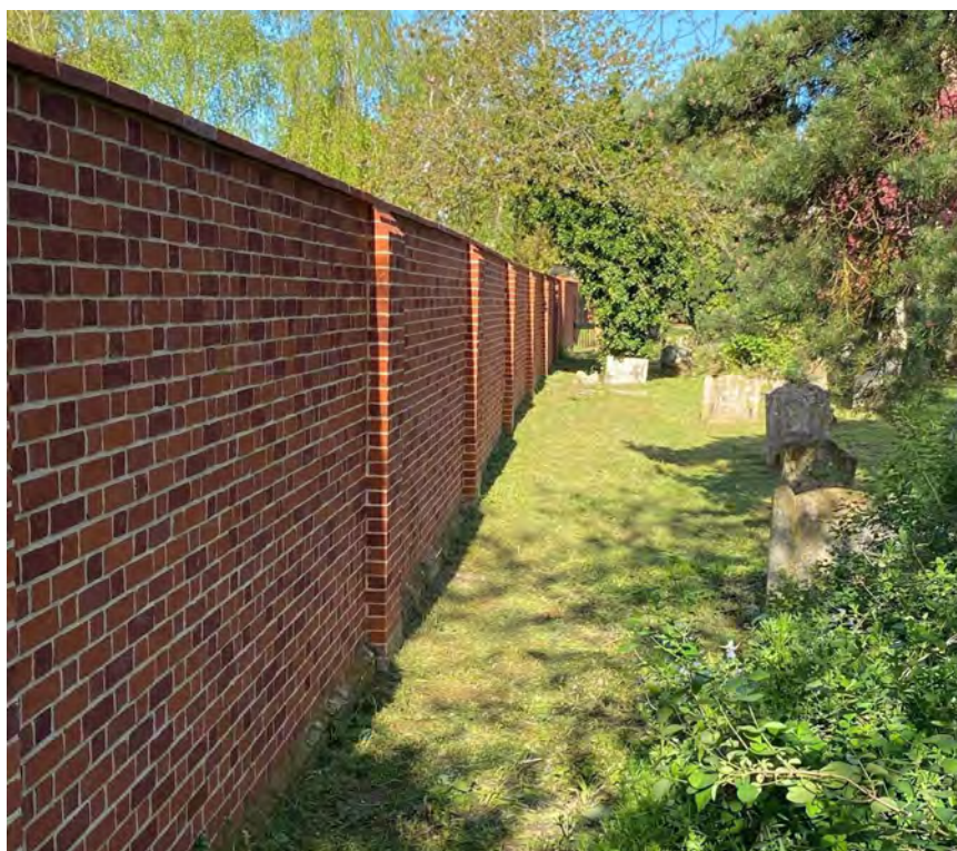
A new wall constructed using lime mortar (Wickham Market).
