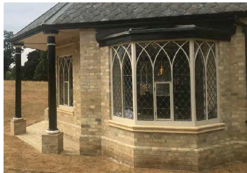
Plinths protrude from the base of a wall on a building extension (Sibton Park Gate Lodge). (Source - Argus Hardy)
