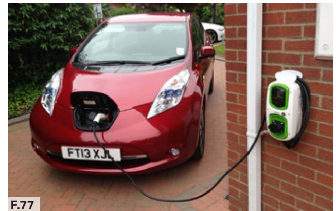
Figure 77: Example of off-road mounted car charging points.
