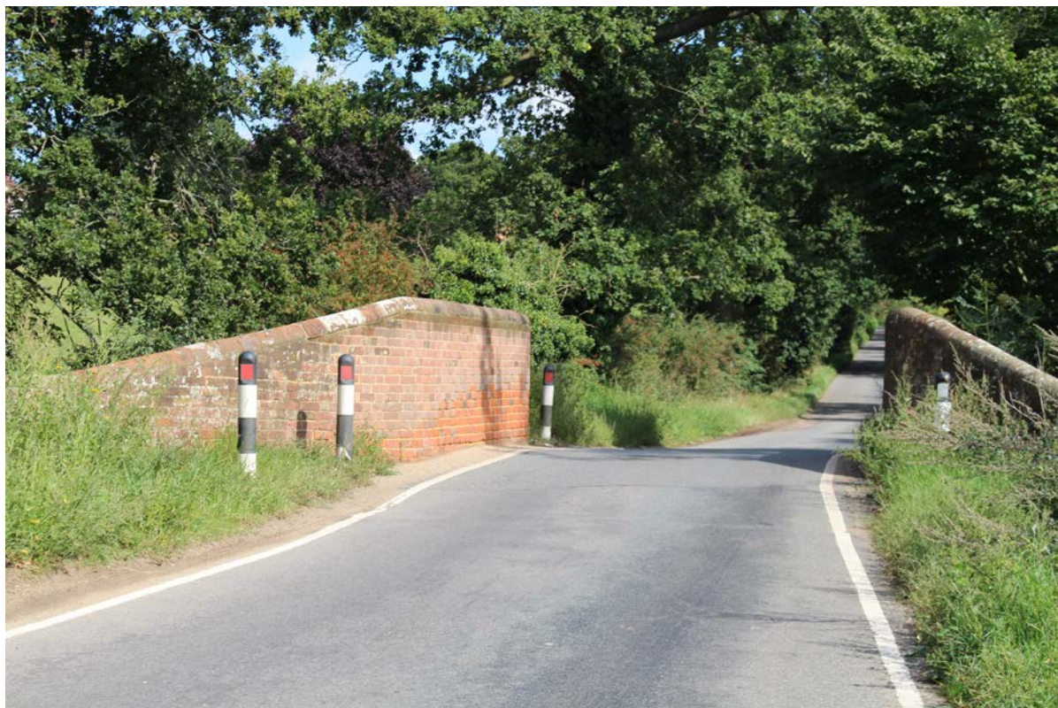
Boot Street bridge
