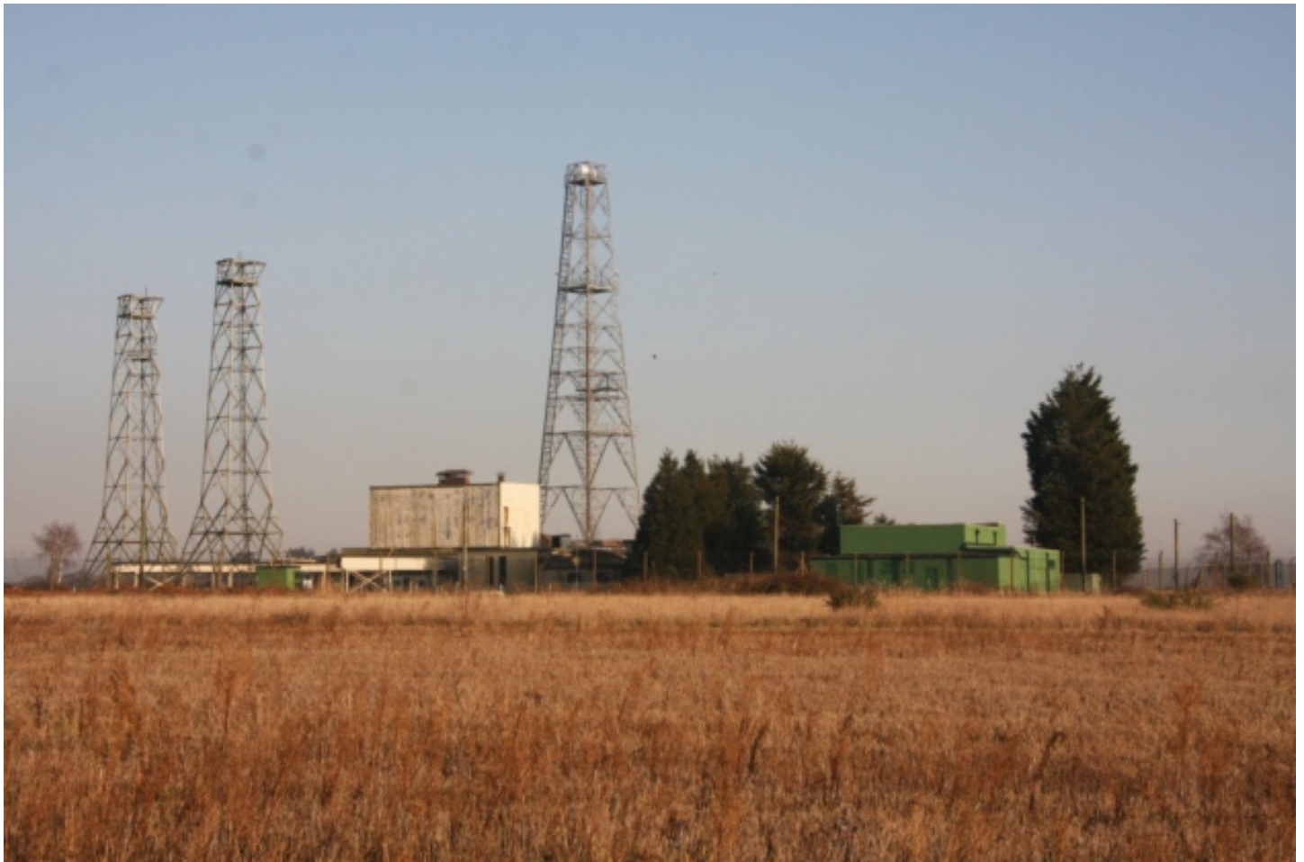
The towers at the site of Suffolk Aviation Heritage Museum in Kesgrave. Picture: CONTRIBUTED
